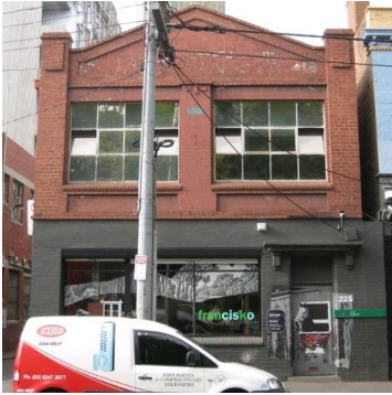
Figure 3. 225-227 Queensbury Street, Carlton, built in 1923.
