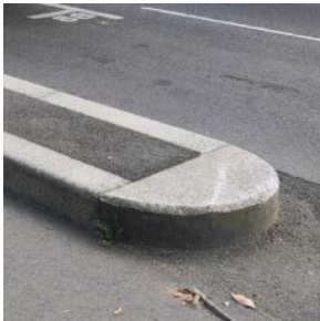
Concrete separator island
