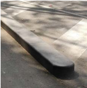
Concrete separator kerb
