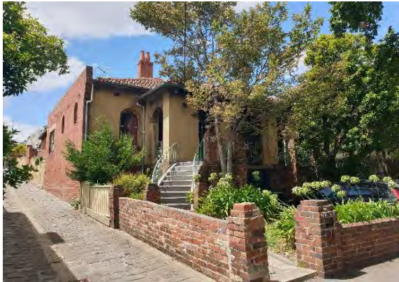
Figure 535. 98 and 98A Flemington Road. (Source: GML, 2022)
