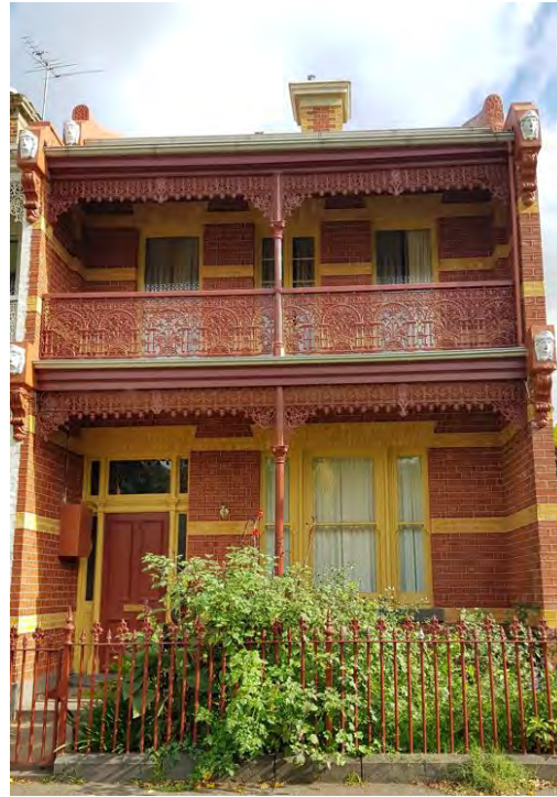
Figure 468. View of the primary eastern elevation of 549 Royal Parade. (Source: GML Heritage, 2022)
