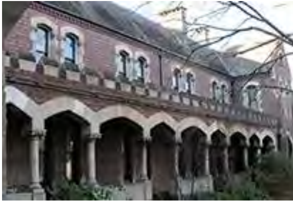
Figure 345. Clarke Building, Trinity College. (Source: Trinity College)
