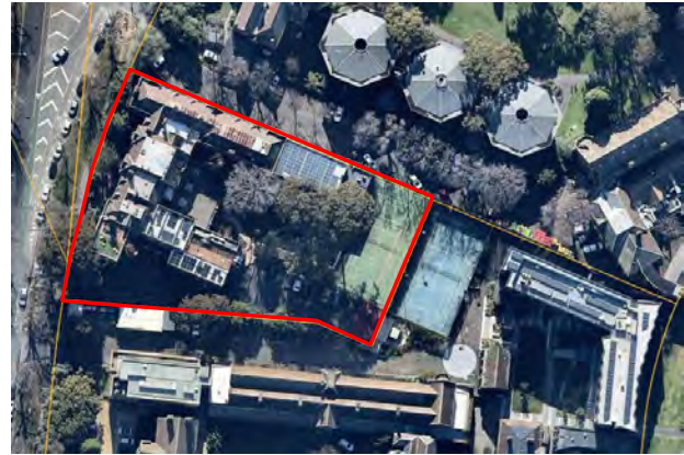
Figure 344. Aerial view of Janet Clarke Hall (denoted in red outline). (Source: Nearmap, with GML overlay)
