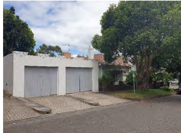
Figure 491. 30–32 Manningham Street from St Georges Grove. (Source: GML 2022)
