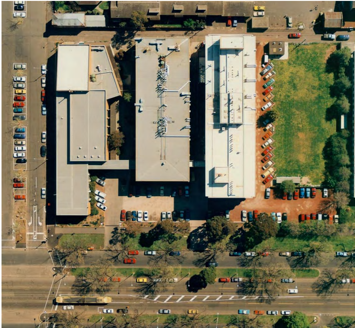
Figure 446. Aerial view of the Victorian College of Pharmacy in 1995. (Source: Monash University Archives)
