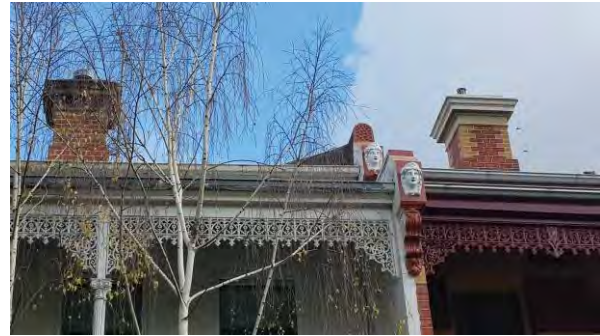
Figure 470. Detail showing decorative fascias, corbels and Italianate chimneys between Nos 547 and 549. (Source: GML Heritage, 2022)
