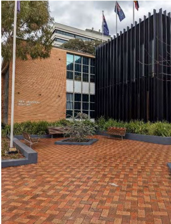
Figure 24. Sissons Building (north elevation) showing the contemporary addition and obstruction to the curtain wall. (Source: GML)
