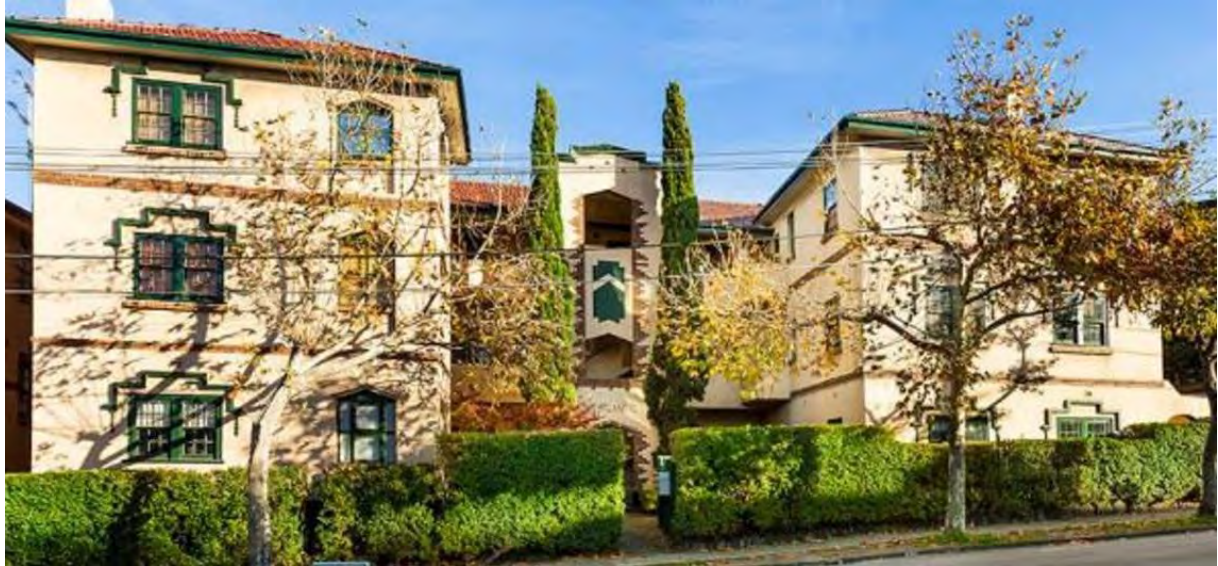
Figure 426. The Atlantic, 101 Barkly Street, St Kilda. (Source: City of Port Phillip via Hermes Orion)
