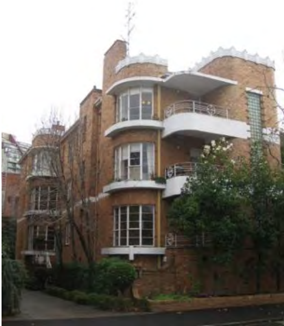
Figure 367. 19–29 Adams Street in South Yarra, built in 1938. (Source: CoMMaps)
