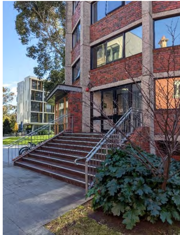
Figure 333. Ida Scheps Wing main entrance. (Source: GML, August 2022)
