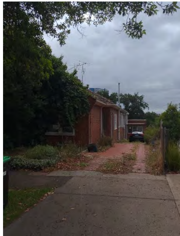
Figure 494. 9 St Georges Grove, Parkville. (Source: GML 2022)
