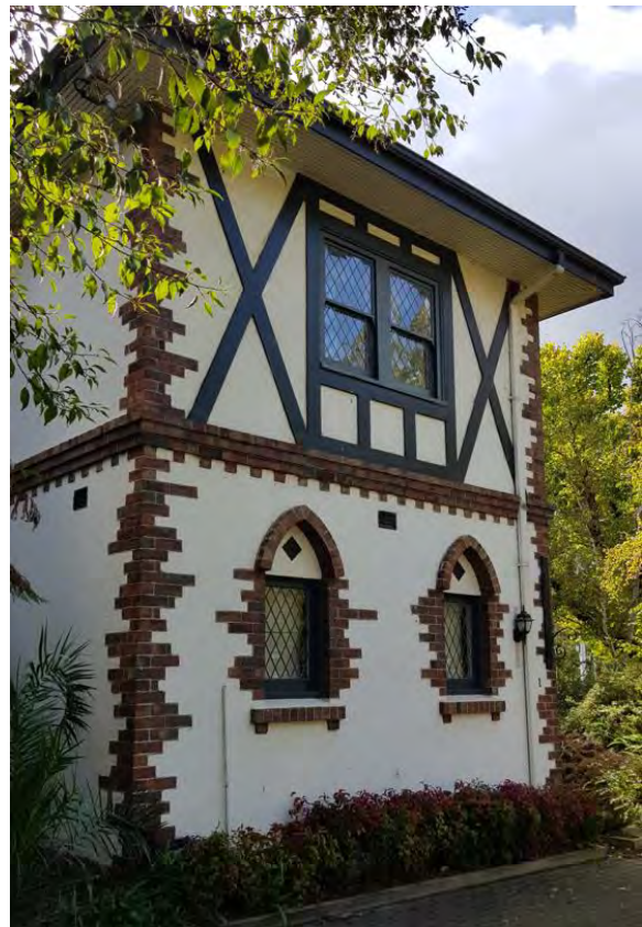
Figure 421. Detail showing a typical elevation with half timbering, and arched brickwork. (Source: GML Heritage, 2022)
