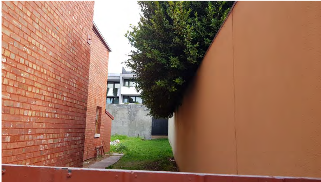
Figure 473. View along the access path towards the rear communal area, with the northern elevation of No. 549 and its rear wing. (Source: GML Heritage, 2022)
