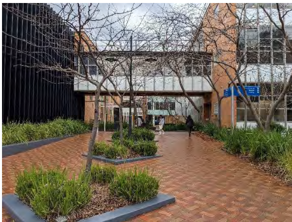
Figure 19. View of the bridge connecting the Sissons and Scott buildings. (Source: GML)
