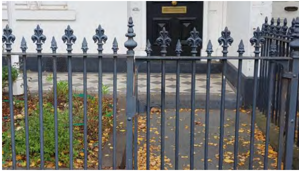
Figure 469. Detail showing the palisade fence, and tiled floor of the verandah at No. 543. (Source: GML Heritage, 2022)
