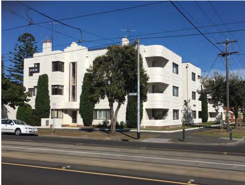
Figure 407. 109 Nimmo Street, Middle Park, built in 1937. (Source: Hermes Orion 198852)
