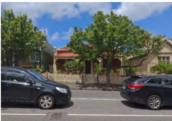
Figure 529. 10–12 Church Street. (Source: GML, 2022)
