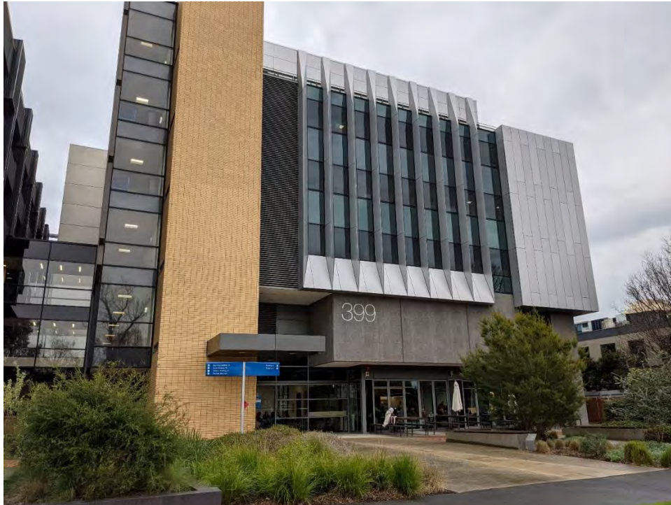
Figure 38. New building at 399 Royal Parade, completed in 2007. (Source: GML)
