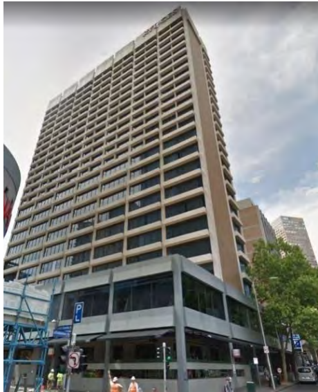
Figure 459. Former Bryson Centre, 174–192 Exhibition Street, Melbourne (HO1332 City of Melbourne). (Source: GML, 2020)
