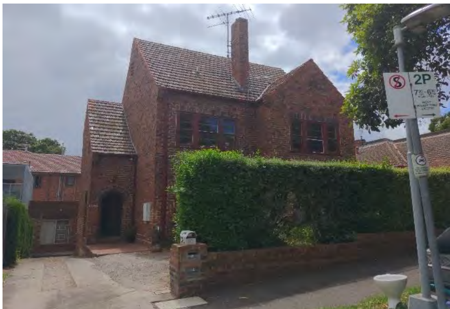
Figure 492. 1–3 St Georges Grove, Parkville. (Source: GML 2022)
