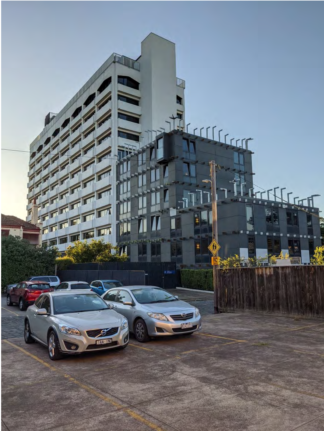
Figure 383. View of the rear of the Former Zebra Motel from Mile Lane. (Source: GML, February 2023)
