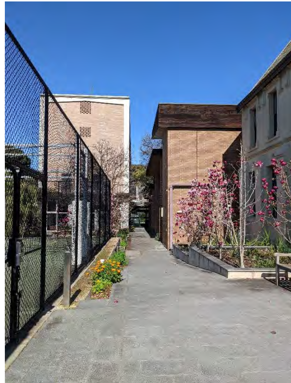
Figure 325. North side of the Samuel Wadham Wing showing the rear of the Dining Hall. (Source: GML, August 2022)
