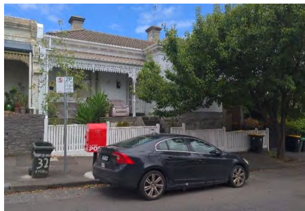
Figure 530. 32 Church Street. (Source: GML, 2022)
