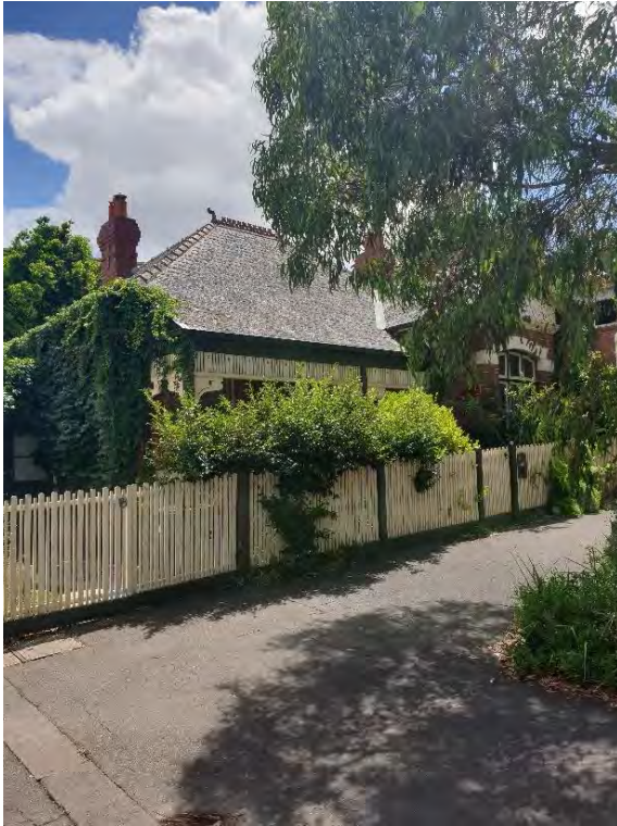
Figure 533. 25–29 Southgate Street. (Source: GML, 2022)
