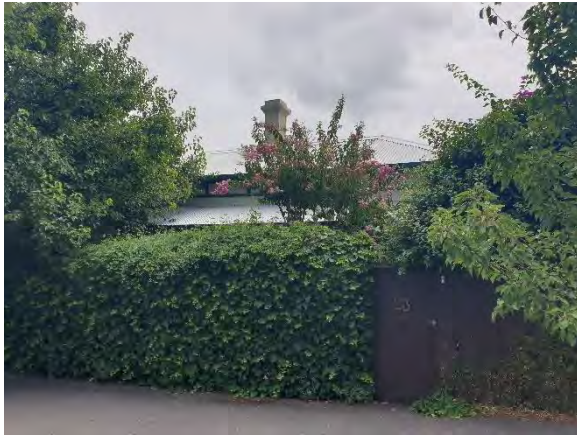
Figure 527. 21–25 Church Street. (Source: GML, 2022)
