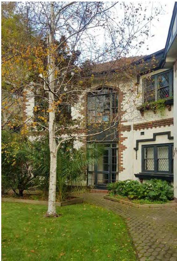
Figure 420. Detail showing the rear wing facing towards the integrated courtyard garden. (Source: GML Heritage, 2022)
