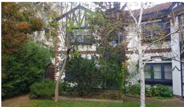
Figure 416. A view toward the eastern-facing elevation, which constitutes the rear of the J-shape. (Source: GML Heritage, 2022)
