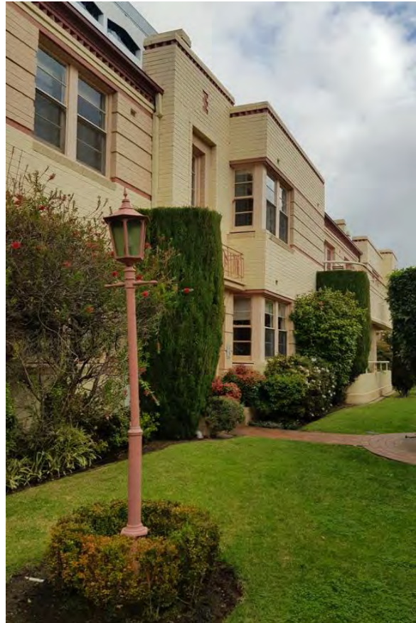
Figure 402. Detail of a projecting bay in the central courtyard showing a parapet. (Source: GML Heritage, 2022)
