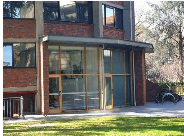
Figure 335. View of former annexe area. (Source: GML, August 2022)
