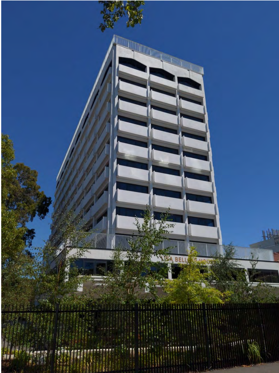
Figure 380. Former Zebra Motel, 303–309 Royal Parade, Parkville. (Source: GML, January 2022)
