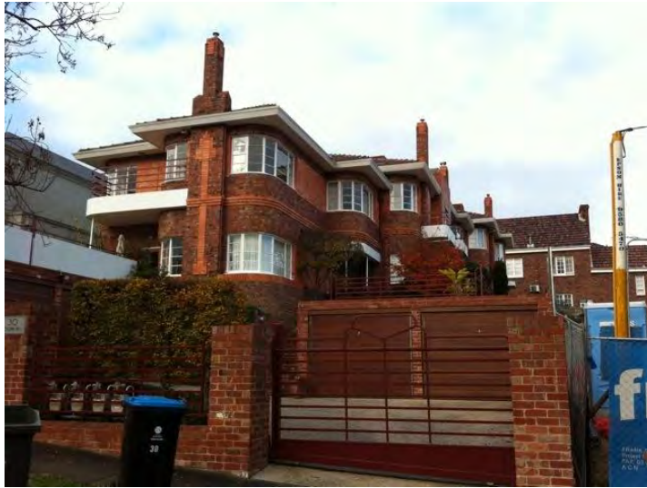
Figure 366. Eden Kyle Flats at 30 Verdant Avenue, Toorak, built in 1939. (Source: Hermes Orion, 165704)
