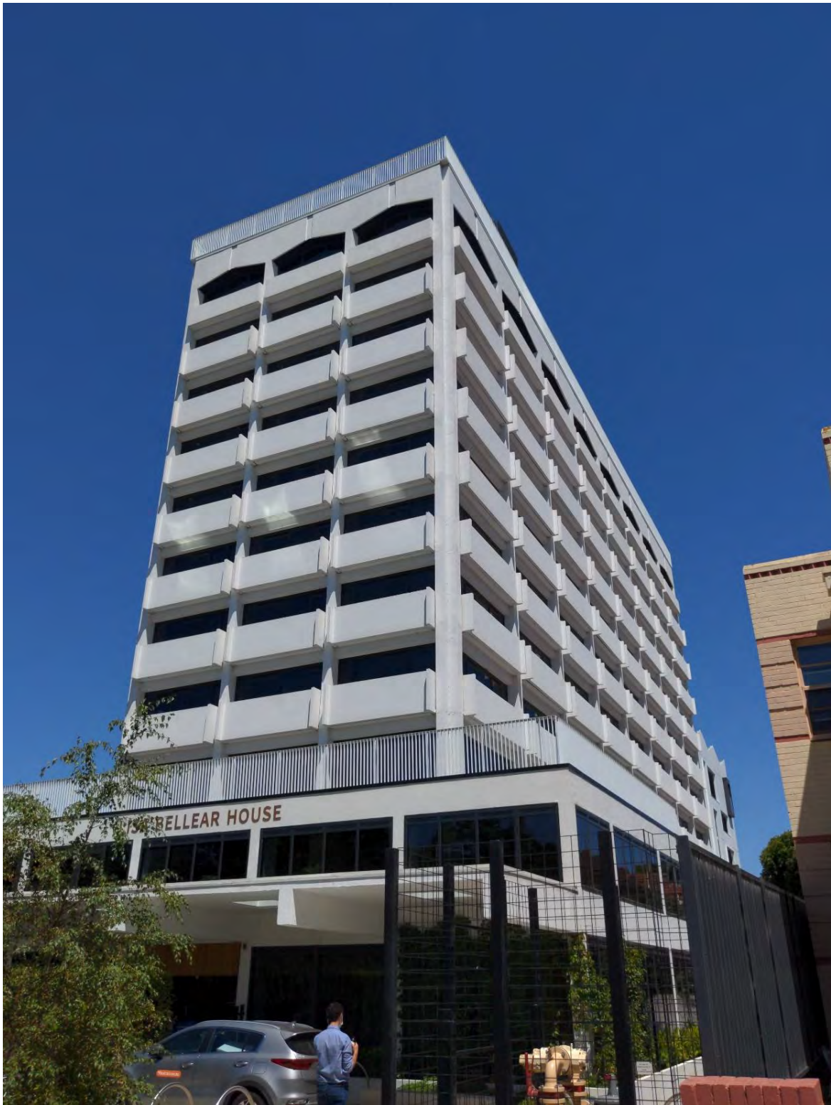
Figure 382. Former Zebra Motel, 303–309 Royal Parade, Parkville. (Source: GML, January 2022)
