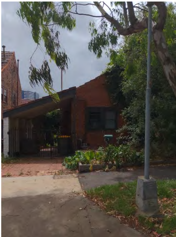
Figure 493. 7 St Georges Grove, Parkville. (Source: GML 2022)
