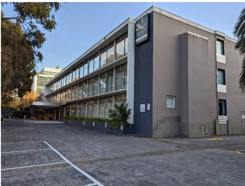
Figure 456. The principal façade at the former Motel Parkroyal, showing the narrow vertical window additions to the north side of the building. (Source: GML, 2022)
