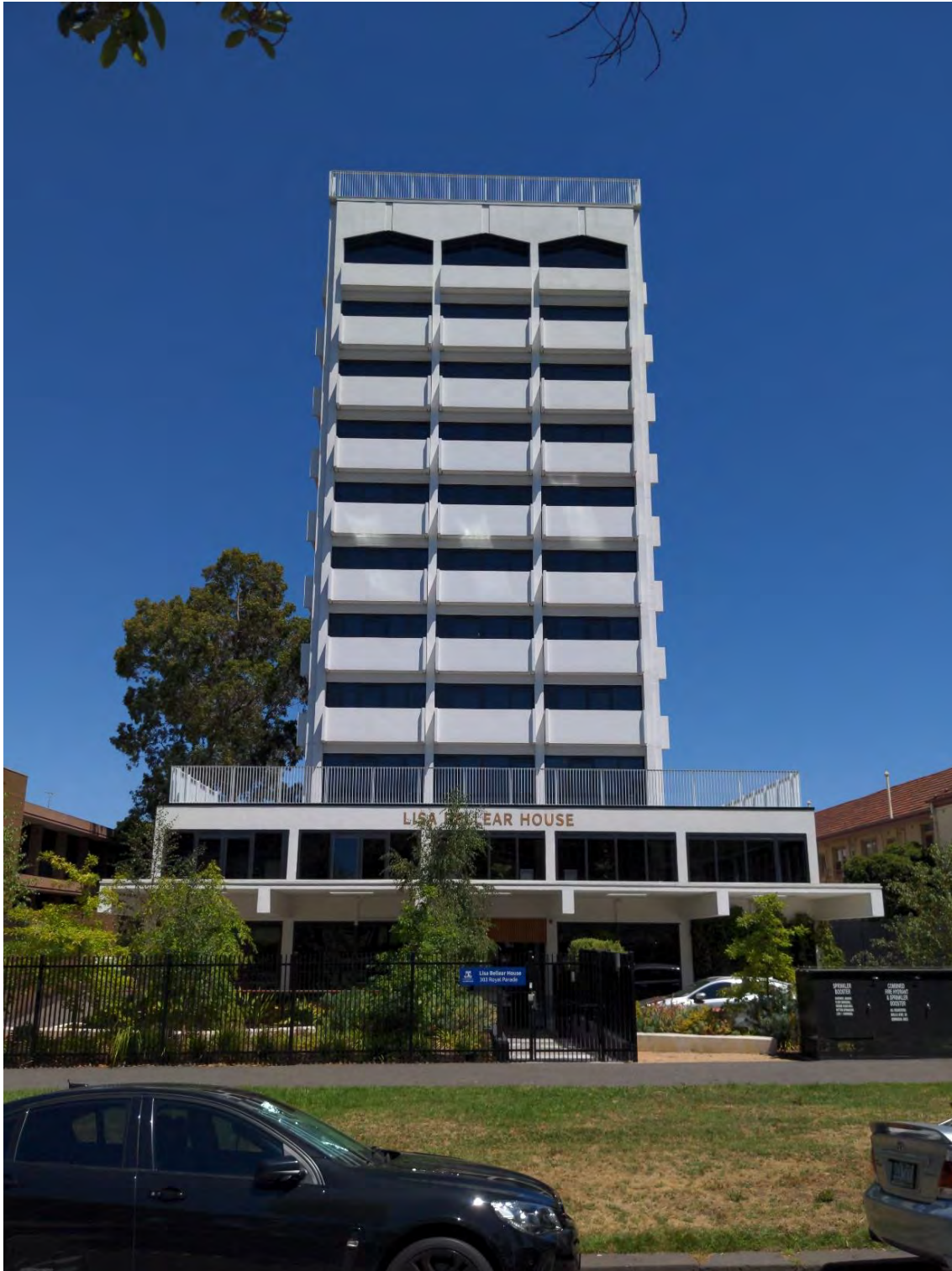
Figure 381. Former Zebra Motel, 303–309 Royal Parade, Parkville. (Source: GML, January 2022)
