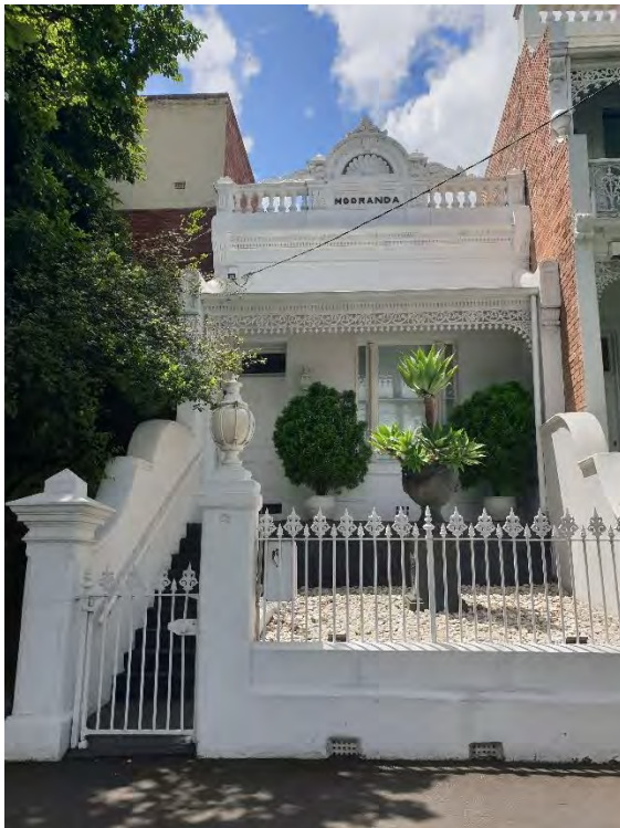
Figure 531. 78 Flemington Road. (Source: GML, 2022)
