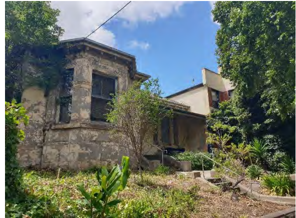
Figure 528. 80–84 Flemington Road. (Source: GML, 2022)
