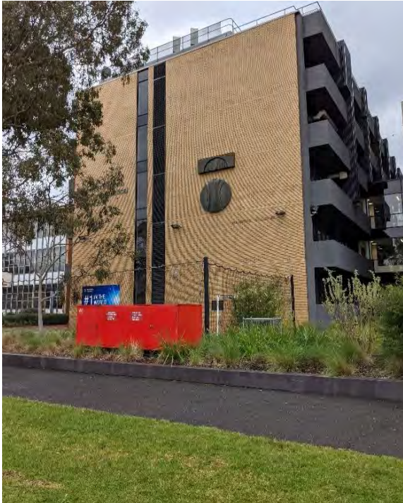
Figure 34. View of the primary (east) elevation of the Manning Building from Royal Parade. (Source: GML)
