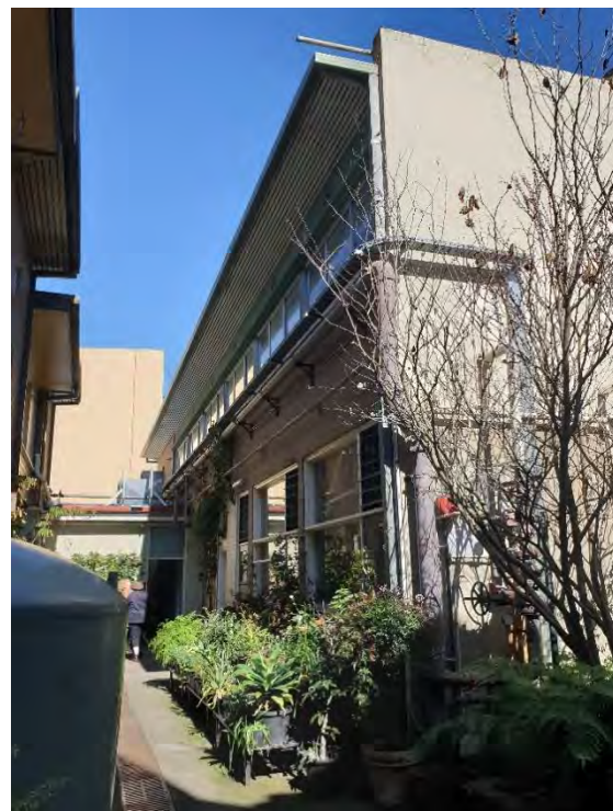
Figure 330. View of the West Wing. (Source: GML, August 2022)
