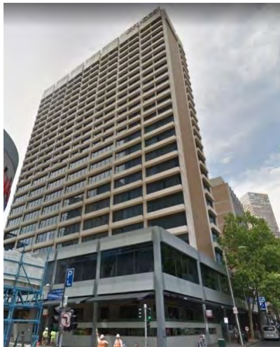
Figure 386. Former Bryson Centre, 174–192 Exhibition Street, Melbourne. (Source: Context)
