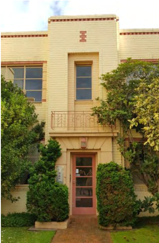
Figure 399. Detail of the primary entrance to the rear wing showing the door surrounds, Juliet balcony and parapet. (Source: GML Heritage, 2022)
