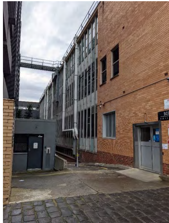
Figure 23. Scott Building (north elevation) when viewed from Mile Lane. (Source: GML)
