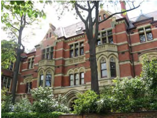
Figure 343. Janet Clarke Hall. (Source: Heritage Victoria)
