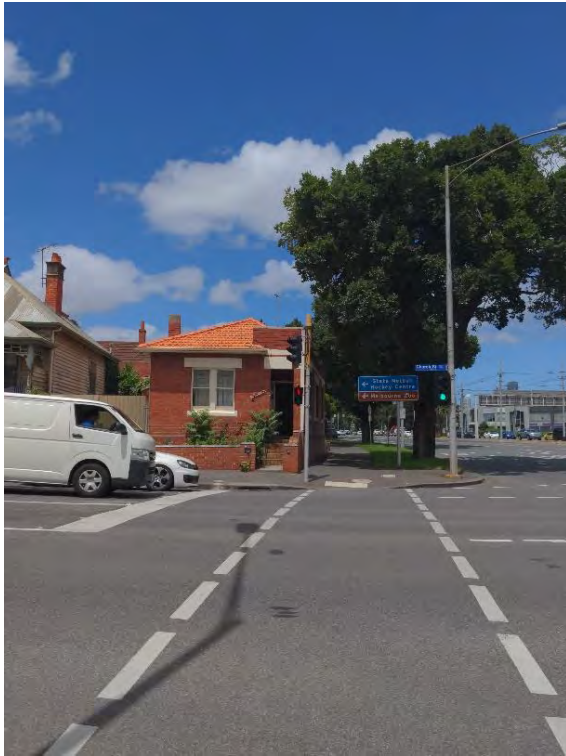
Figure 537. 2–4 Church Street. (Source: GML, 2022)
