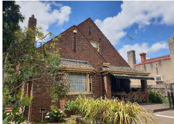
Figure 536. 130–132 Flemington Road. (Source: GML, 2022)
