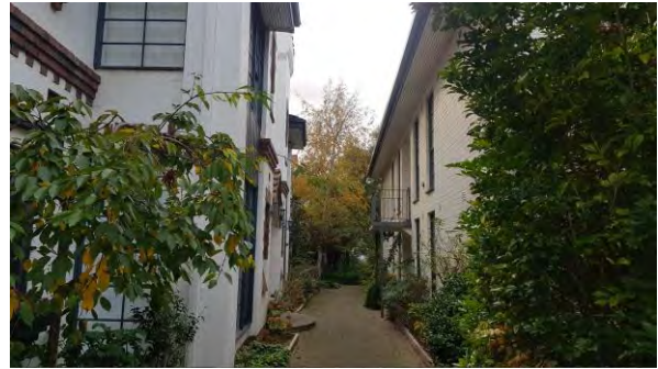
Figure 419. A view showing the central pathway, facing west. (Source: GML Heritage, 2022)
