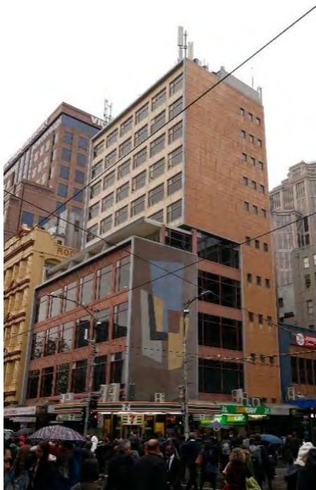
Figure 458. Former Hosie's Hotel, 1–5 Elizabeth Street, Melbourne (HO1327 City of Melbourne). (Source: GML, 2020)
