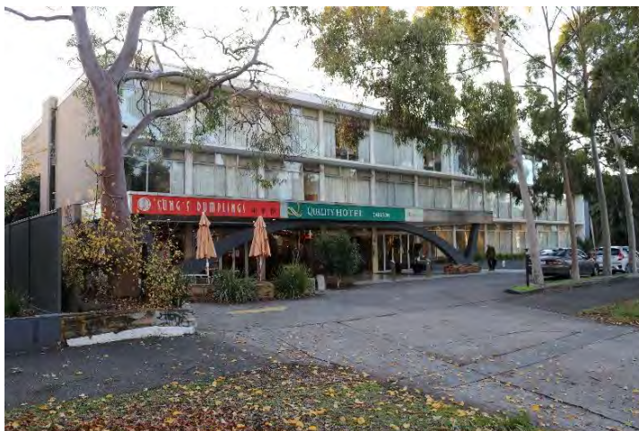
Figure 385. Former Motel Parkroyal, 441 Royal Parade, Parkville. (Source: GML 2022)
