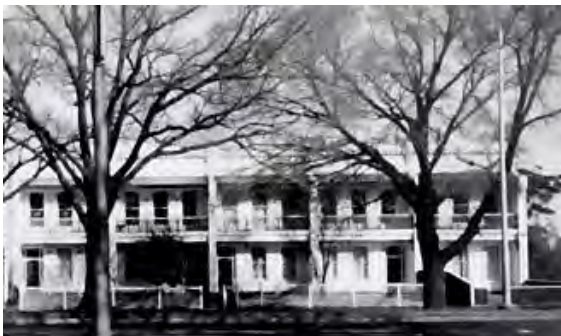
Figure 477. A view of Park Terrace, Parkville, c1975. (Source: Victorian Heritage Register)
