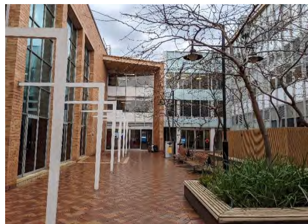
Figure 31. View of asymmetrical volume (Sissons Building, left) and contemporary addition (Scott Building, right). (Source: GML)
