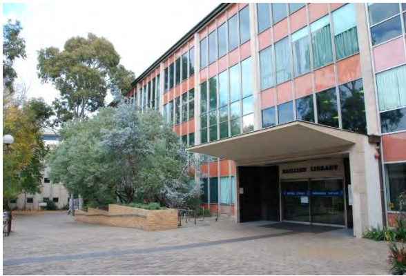
Figure 44. The Baillieu Library, designed by John FD Scarborough 1951–54, constructed in 1957–59. (Source: VicScreen)
