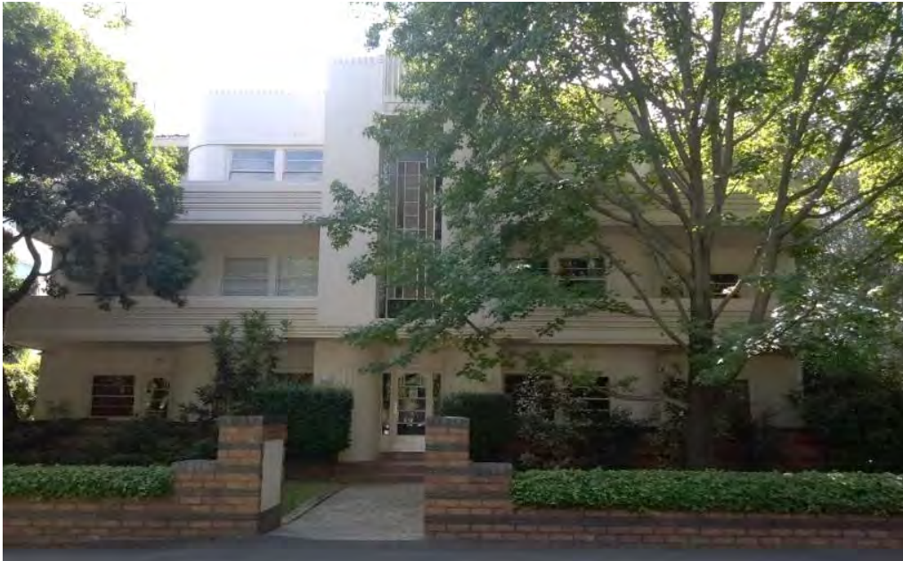
Figure 406. Kia Ora, 447–453 St Kilda Road, South Yarra, built in 1936–37. (Source: GML Heritage, 2021)
