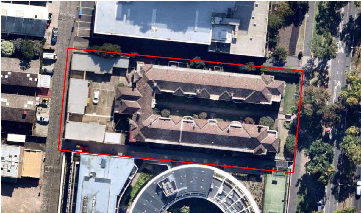
Figure 355. Aerial view of the site in 2022, showing the building, its central courtyard, and garages and shedding to the west. The boundary of the site is approximately indicated in red. (Source: Nearmap, 2022, with GML overlay)
