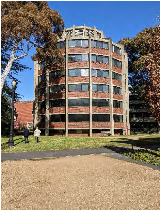
Figure 332. Scheps Wing looking south. (Source: GML, August 2022)
