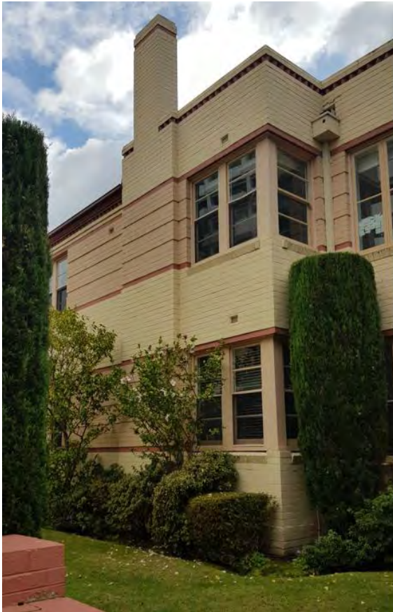
Figure 401. Detail of a projecting bay in the central courtyard showing a chimney. (Source: GML Heritage, 2022)
