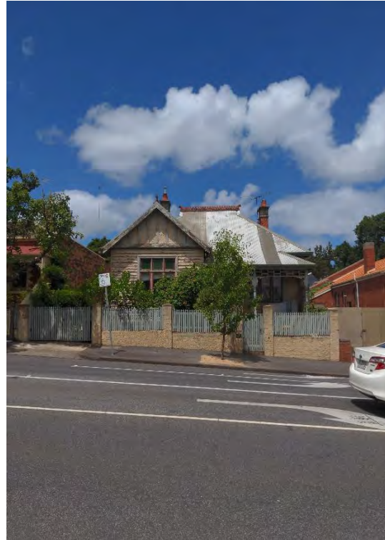
Figure 534. 6–8 Church Street. (Source: GML, 2022)
