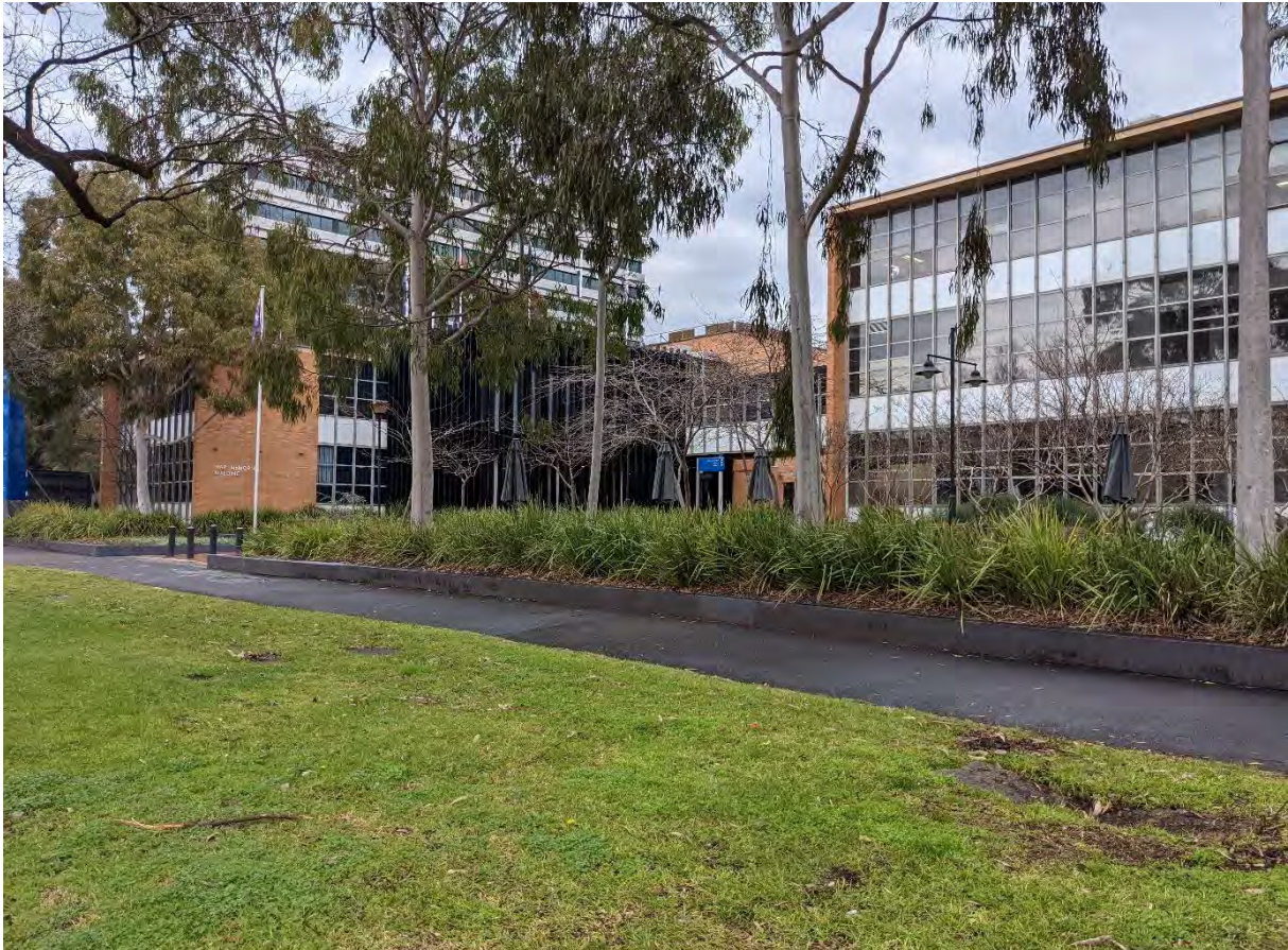
Figure 21. Sissons and Scott Buildings when viewed from Royal Parade. (Source: GML)
