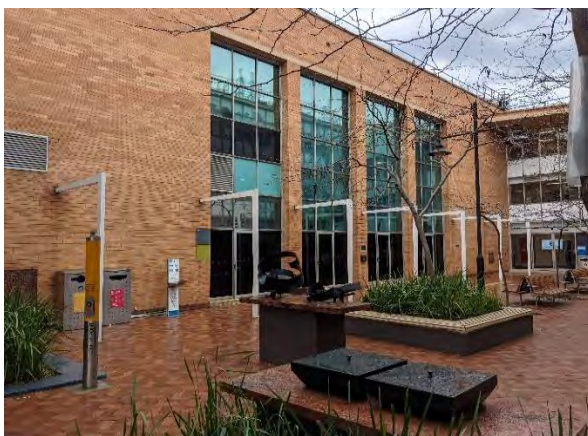
Figure 30. Sissons Building (north elevation) showing the white frames and Acrux sculpture by Lenton Parr in the foreground. (Source: GML)
