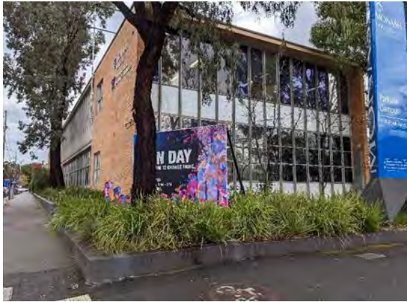
Figure 17. Primary (east) façade of the Sissons Building when viewed from the corner of Walker Street and Royal Parade. (Source: GML)
