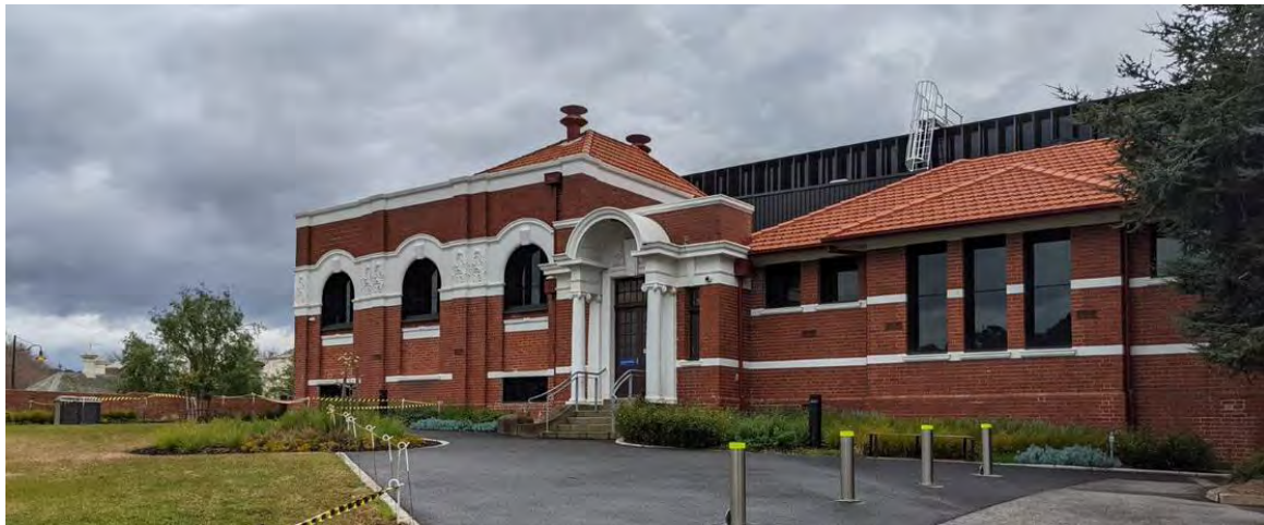
Figure 514. 1908 Veterinary College building. Note the original window frames have been replaced and a large (black) extension has been added to its rear. (Source: GML Heritage, 2022)
