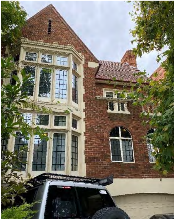
Figure 429. Tudor Lodge, 180–182 Toorak Road West, South Yarra. (Source: Context, 2021)
