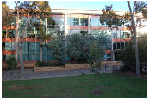
Figure 45. The Baillieu Library. (Source: VicScreen)
