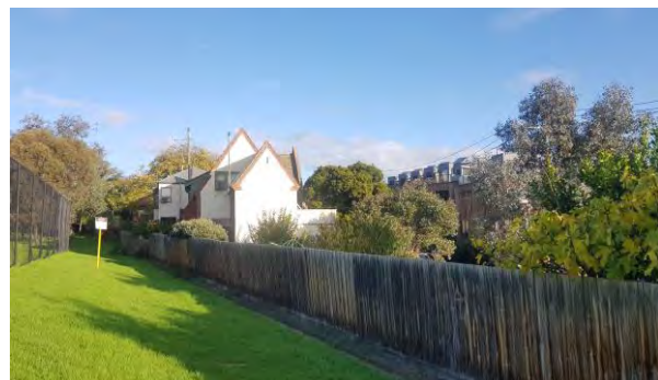
Figure 47. View showing the eastern elevation of the property, looking southwest. (Source: GML Heritage, 2022)
