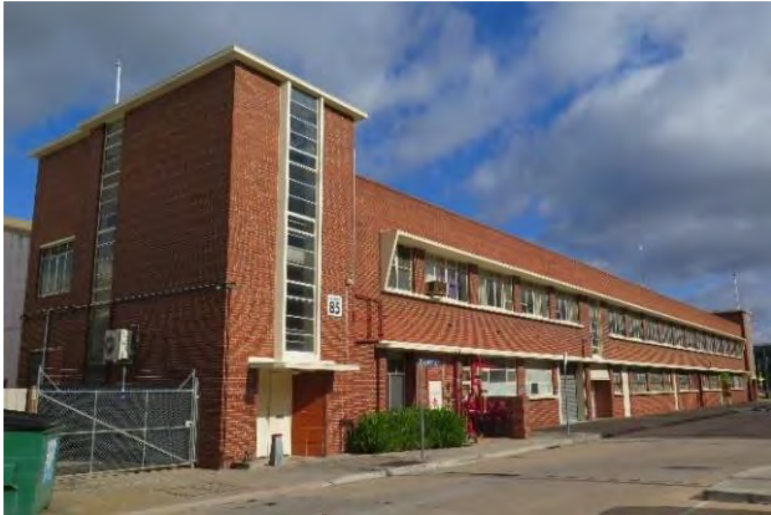
Figure 181. The Beaufort Building (Building 85). (Source: GML Heritage, 2019)
