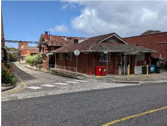
Figure 162. View of the Electrical Maintenance Workshop looking south. (Source: GML, December 2022)
