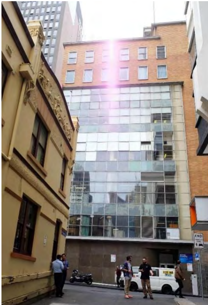
Figure 185. Former Batman Automatic Telephone Exchange, Melbourne. (Source: Context and GJM, 2022)
