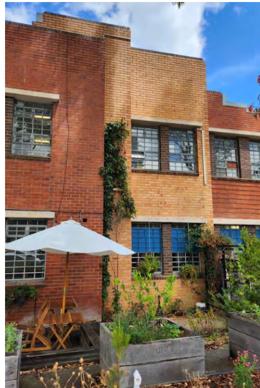
Figure 125. View of the middle bay that originally housed the primary entrance and a stairwell with a vertical statement window. Note the altered openings and removal of the flagpole. (Source: GML, February 2023)
