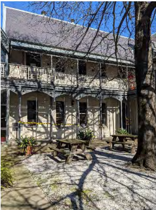
Figure 306. View of the southeast, the 1904–05 addition. (Source: GML, August 2022)
