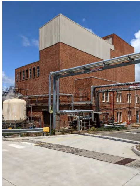
Figure 172. View of the Boiler House (east elevation), showing corrugated metal clad addition. (Source: GML, February 2023)
