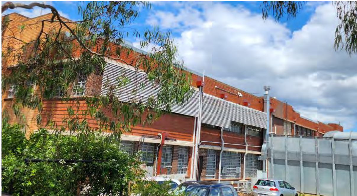
Figure 126. View of the west elevation added with later sunshades and piping. (Source: GML, February 2023)
