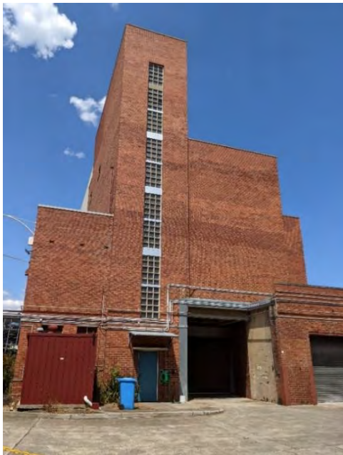
Figure 171. View of the Boiler House (west elevation). (Source: GML, February 2023)
