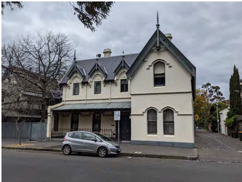
Figure 298. Original 1886–87 section of the building viewed from the corner of Leonard Street and Mile Lane. (Source: GML, August 2022)
