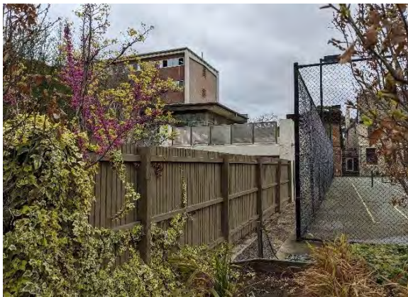
Figure 318. Partial view of the Warden's Residence from Royal Parade. (Source: GML, August 2022)
