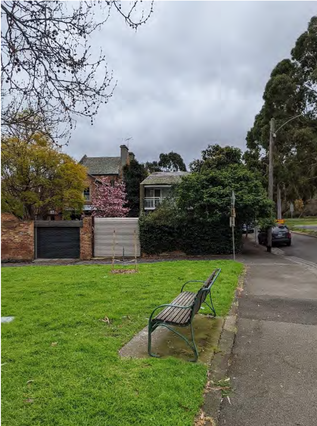
Figure 14. View of the Saunders House from Ievers Reserve. (Source: GML, September 2022)
