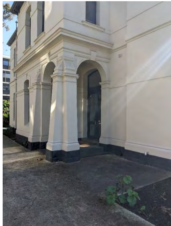
Figure 293. View of southern side porch with buttresses. (Source: GML, August 2022)
