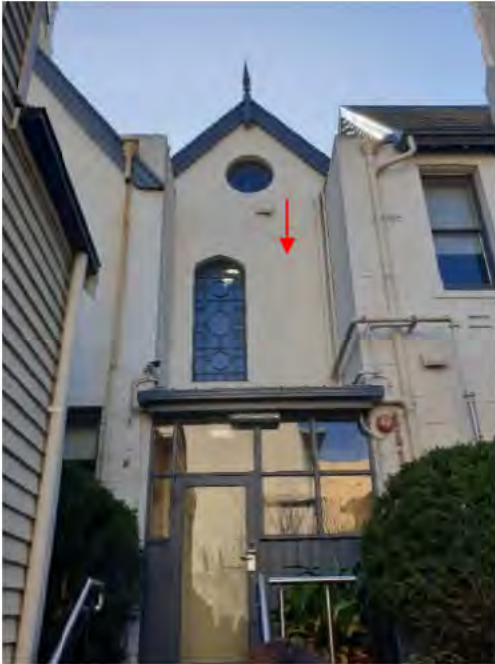
Figure 304. Rear view of the 1904–05 addition. Evidence remains of a window (right; indicated by red arrow) which had likely been removed to accommodate the southeast addition. (Source: GML, August 2022)
