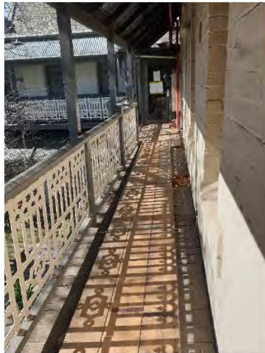
Figure 307. View from the verandah looking east along the 1904–05 addition, with a partial view of the 1907 addition (left). (Source: GML, August 2022)
