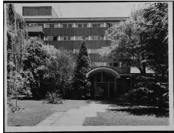
Figure 282. Samuel Wadham Wing. (Source: International House Archives, University of Melbourne)
