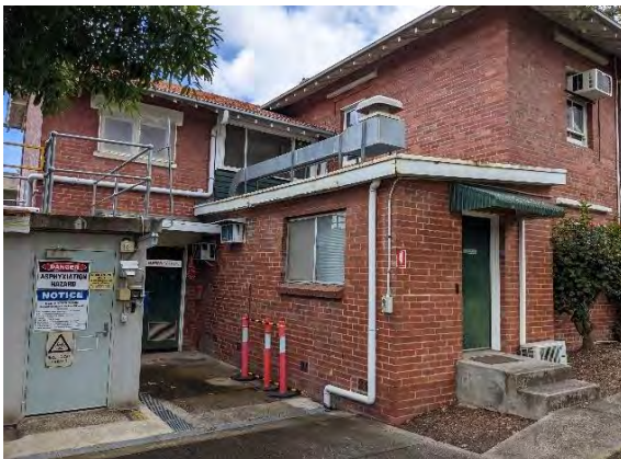
Figure 156. Director's Residence (east elevation). (Source: GML, December 2022)
