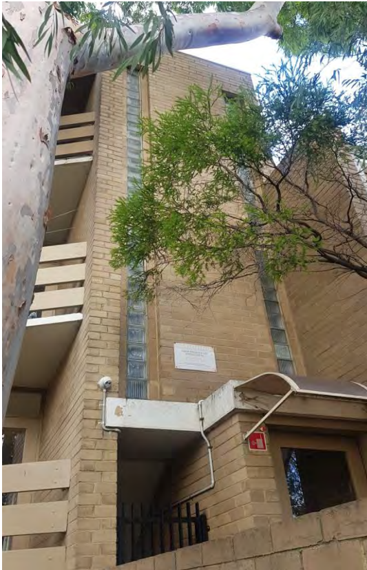
Figure 96. Detail of a stairwell bay with columns of glass bricks. (Source: GML Heritage, 2022)
