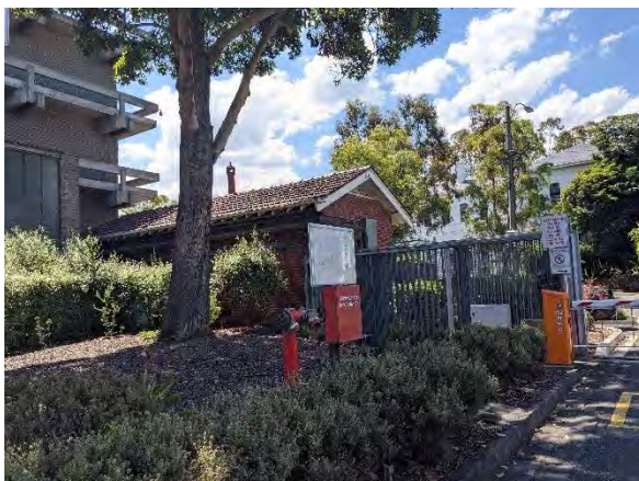
Figure 164. Northern substation. (Source: GML, 2023)
