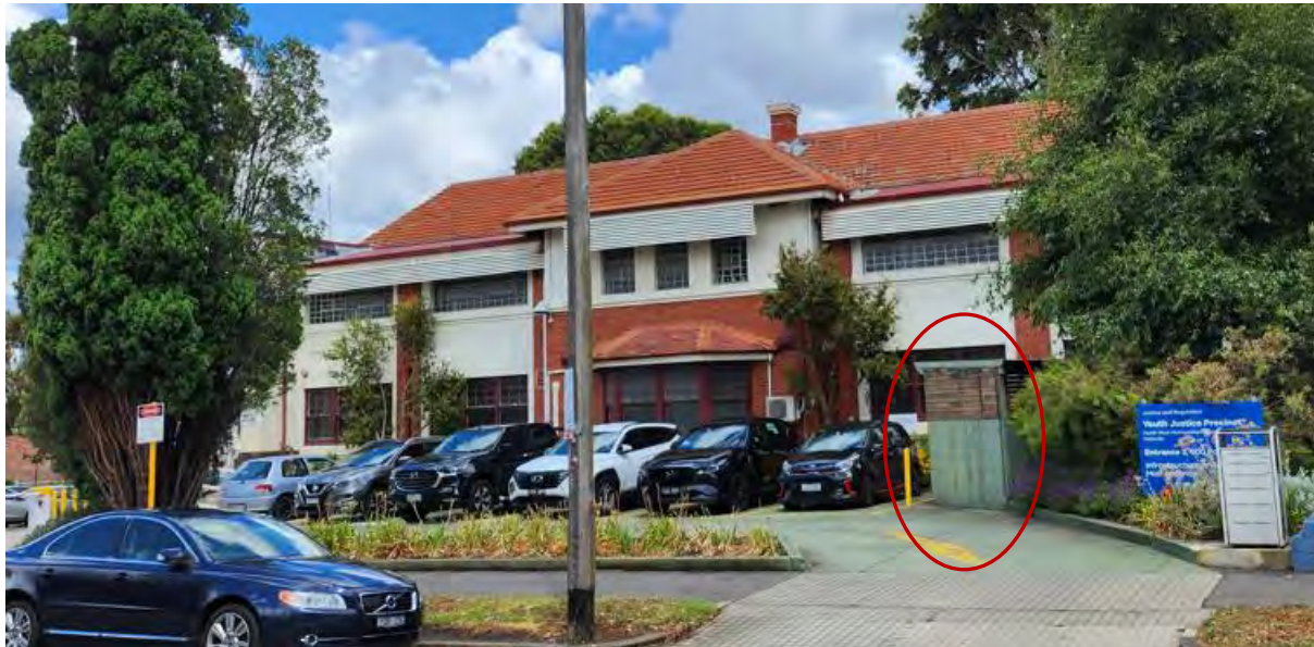
Figure 120. View of the primary elevation of the Administration Building from the northwest. Note the semicircular driveway loop, with a small parking area, and a nature strip. The landscaping on the front setback and the concrete block shed (outlined in red) are recent. (Source: GML, February 2023)
