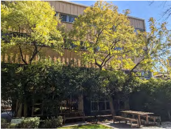
Figure 312. View of Clunies Ross Building (east side). (Source: GML, August 2022)
