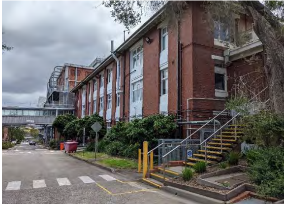
Figure 158. South Block (south elevation) viewed from Fourth Avenue looking west. (Source: GML, December 2022)
