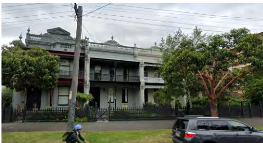
Figure 251. 272–278 The Avenue, Parkville. (Source: GML, 2022)
