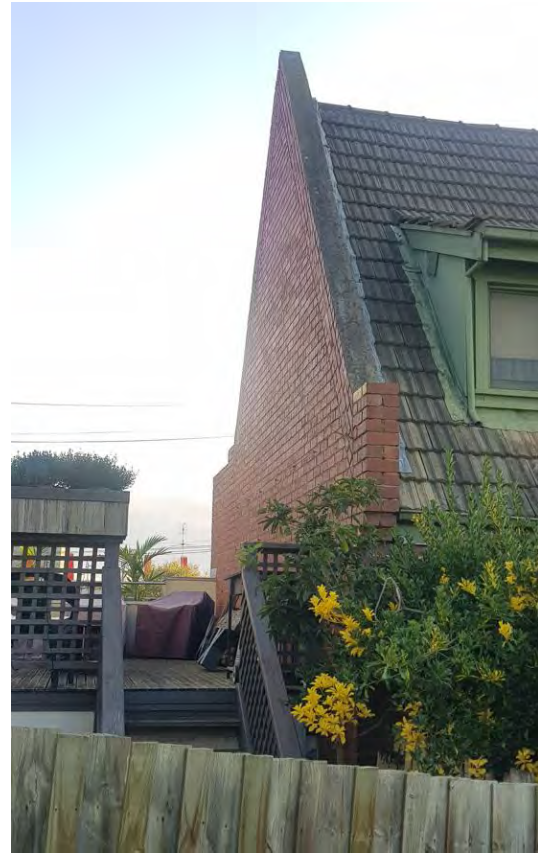
Figure 53. Detail showing the southern elevation and the adjoining deck of the neighbouring property. (Source: GML Heritage, 2022)
