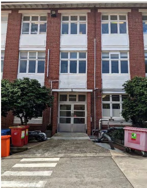
Figure 160. South Block (south elevation) depicting the main entrance from the south (primary) façade. (Source: GML, December 2022)
