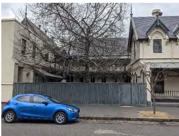
Figure 299. View of the internal courtyard and U-shaped plan of the building additions from Leonard Street. The 1904–05 addition is located at the centre, with the 1907 and 1937 additions situated to the east. (Source: GML, August 2022)
