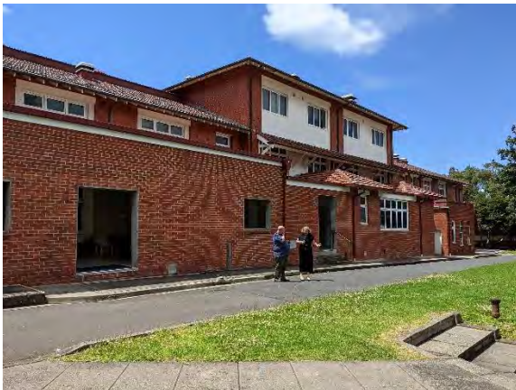
Figure 151. East Block west elevation, showing additions to the northwest area of the building. (Source: GML, December 2022)
