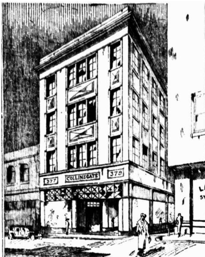
Figure 2. Showing an impression of the subject building in 1925. (Source: Herald 21 October 1925: 16)
