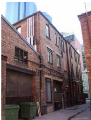
Figure 7. Rear of Union Bond Melbourne Storage Company Ltd, 115-129 King Street constructed 1882.
