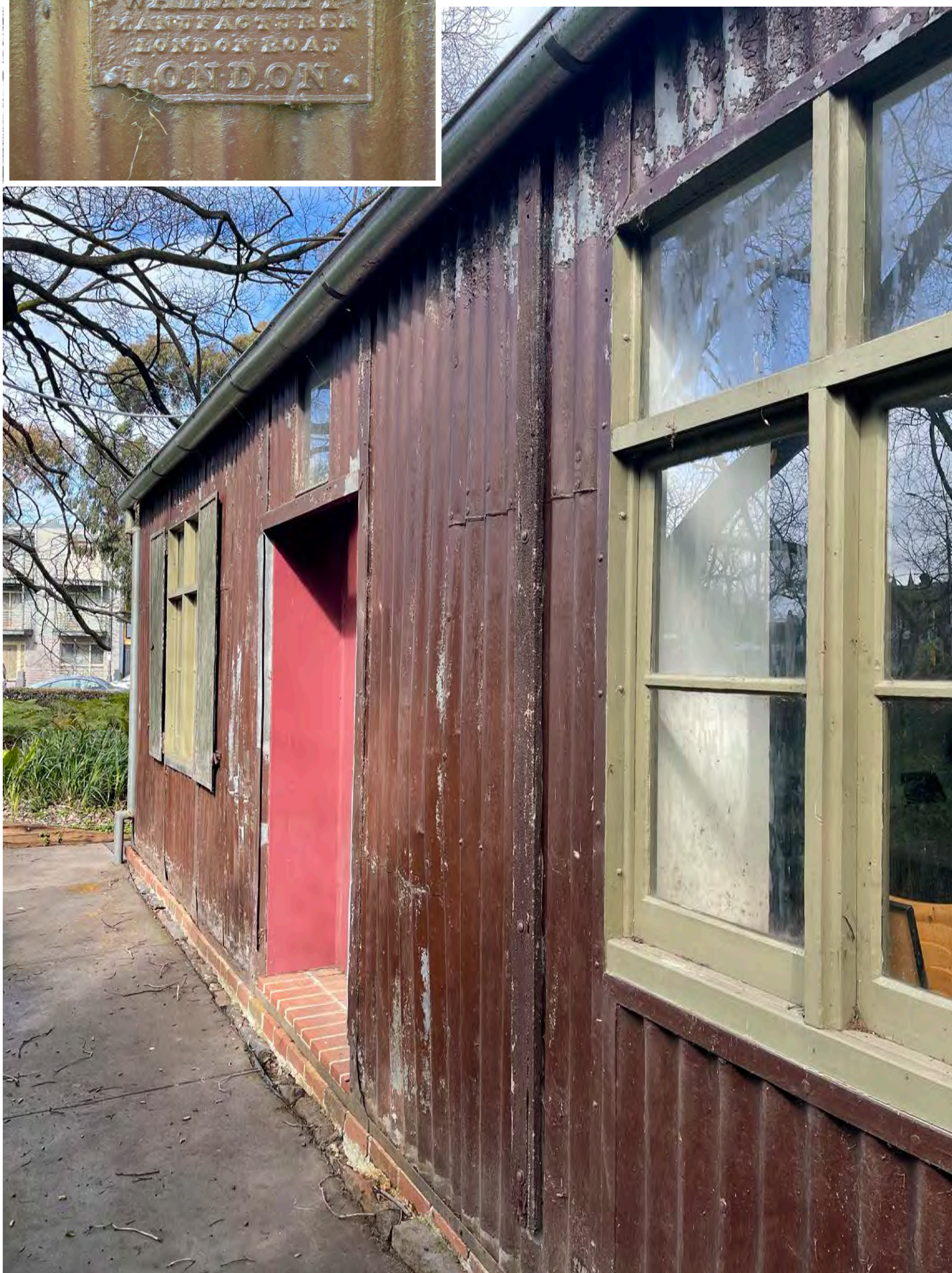
Inset: The manufacturer's plaque. Source: Inset Royal Park Protection Group, retrieved 27/11/23. Main: Walmsley House North elevation, looking towards Gatehouse Street
