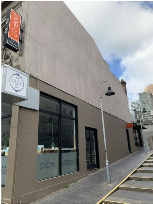
Figure 16 West elevation, showing render finish and new openings along Punch Lane
