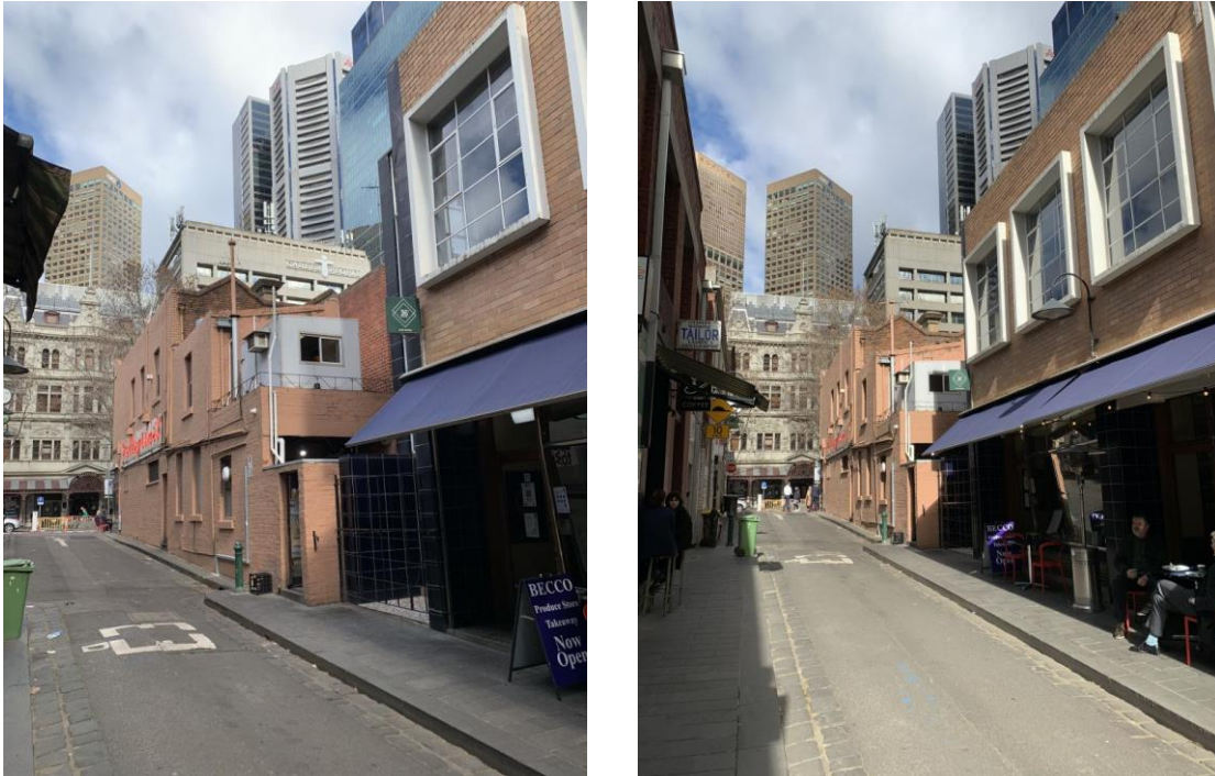
Figure 20 Rear wings and rendered brick chimney visible from Crossley Street
