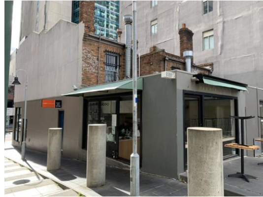
Figure 16 West elevation, showing render finish and new openings along Punch Lane
