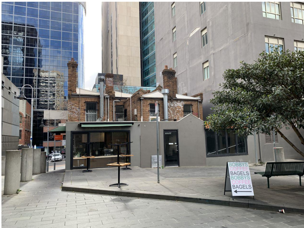
Figure 17 View of the rear wings (south elevation) and the c.2004 single-storey addition to the rear of the subject site
