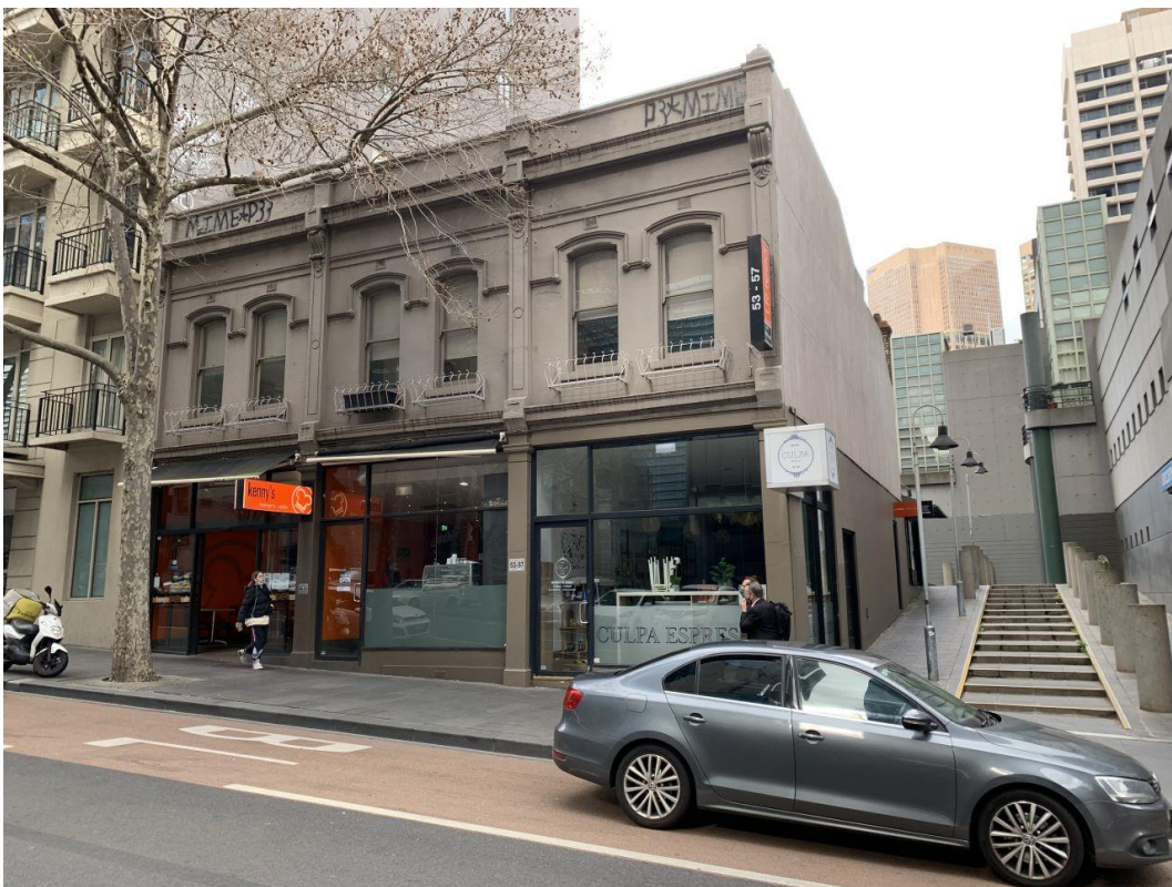
Figure 15 53-57 Lonsdale Street, north and west elevations
