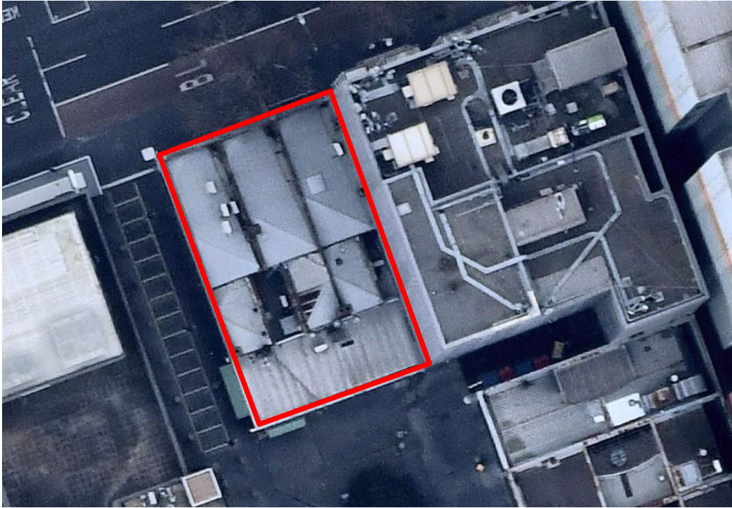
Figure 14 Recent aerial photograph of the subject property (indicated) Source: Nearmap
