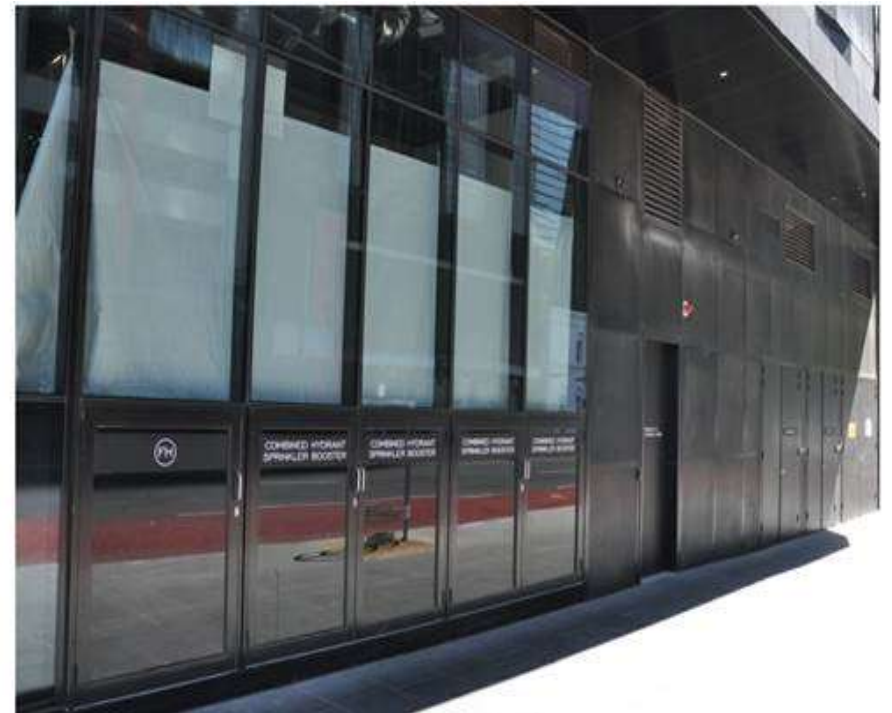
Services located below flood level and poorly designed interface to the public realm results in a blank wall
