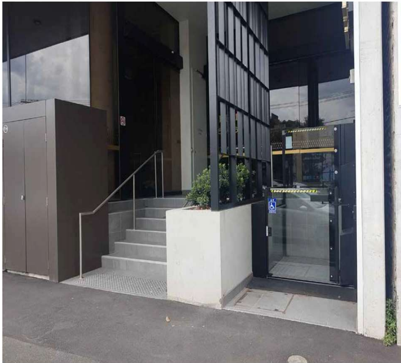
Main building entry recessed from street and concealed by external platform lift and services enclosure
