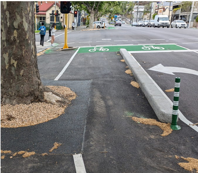
Completed riding lanes at the intersection of Arden Street and Errol Street.
