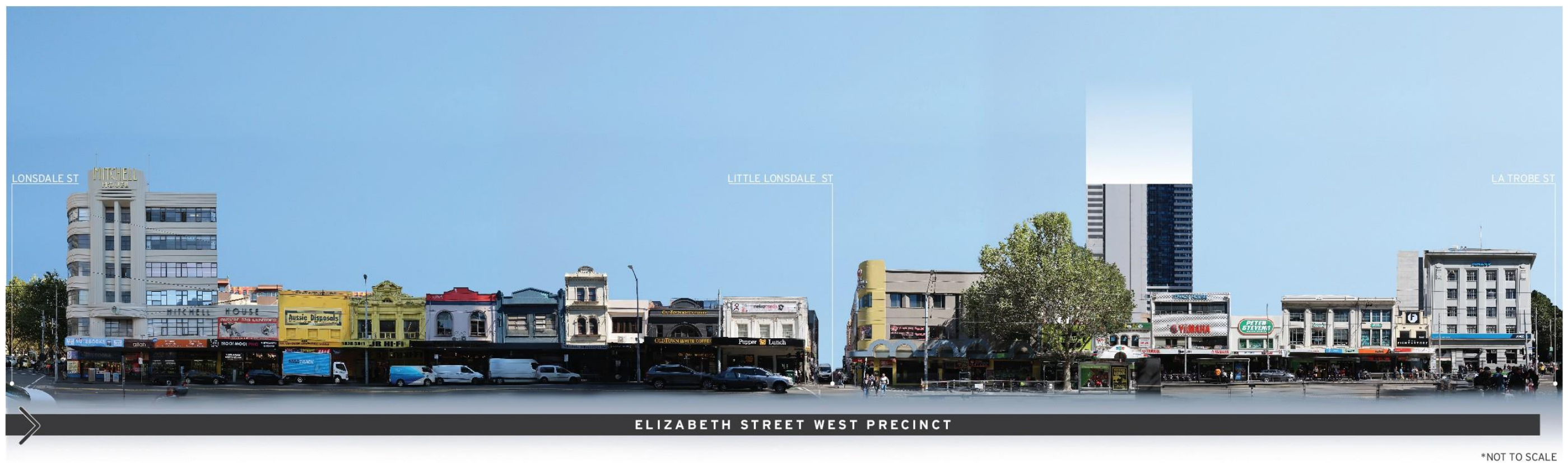
Figure 36 Photo elevation of Elizabeth Street West Precinct showing blocks between Bourke and La Trobe streets
