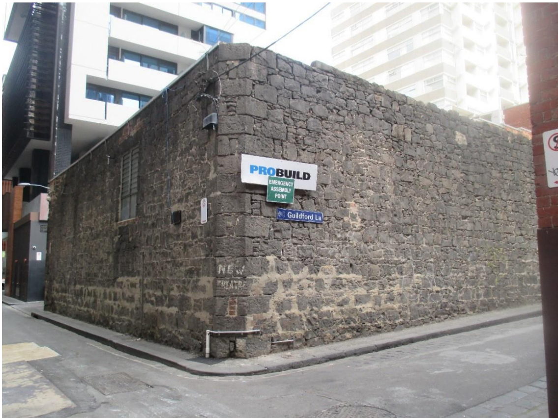
Figure 38 Former Bucks Head Hotel stables, 15 Sutherland Street
