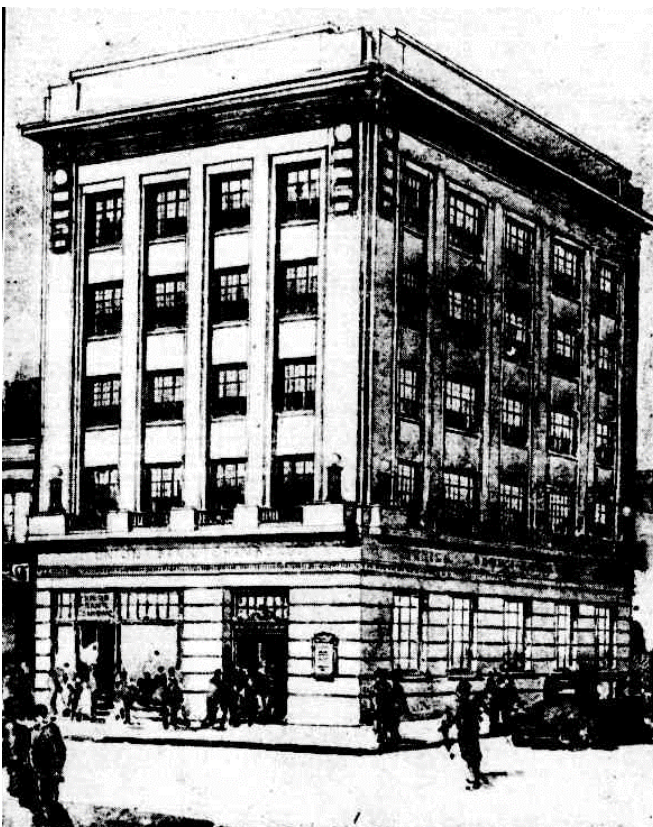
Figure 8 Illustration of new Union Bank at corner of Elizabeth and La Trobe streets Source: Argus , 4 February 1927, p. 15
