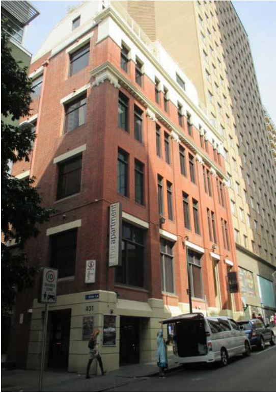
Figure 53 Subject building, looking west
