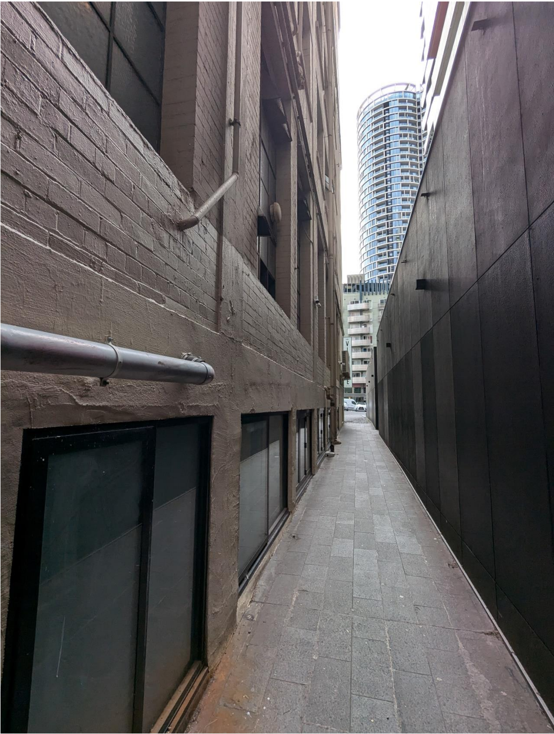
Figure 4: Existing conditions of proposed Benz Lane, looking north
