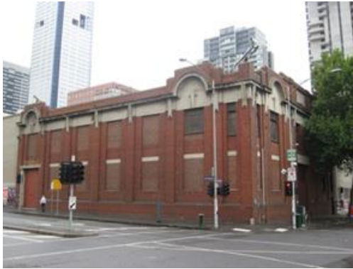
Figure 2. Substation at 651-669 Lonsdale Street constructed 1915.
