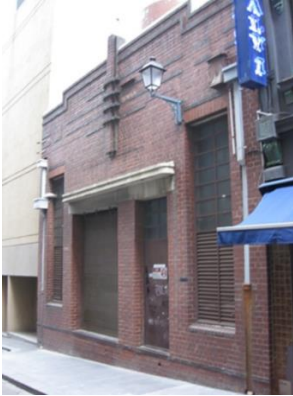
Figure 9. 23-25 George Parade constructed 1938. (Source: Context 2017)
