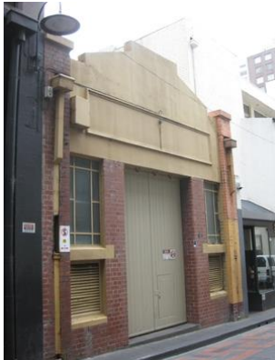
Figure 7. 21 Market Lane, build date unknown.
