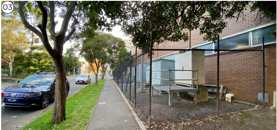
Interface with Substation building and fence
