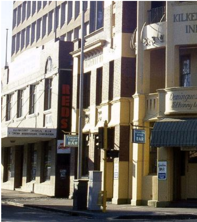
Figure 3. The subject site, to the left-hand side of Kilkeny Inn, with a sign on the cantilevered verandah reading 'Paramount Universal MGM Cinema International Corporation'. (Source: Butler 1982 copyright )
