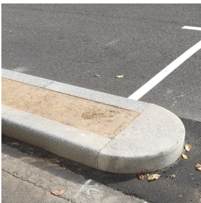
Concrete separator islands
