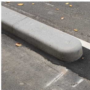
Concrete separator kerbs
