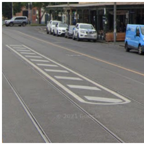
Road narrowing/painted island
