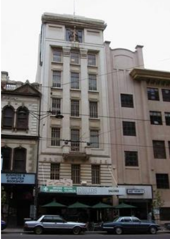
Figure 6. Druids House, 407-409 Swanston Street constructed 1927.
