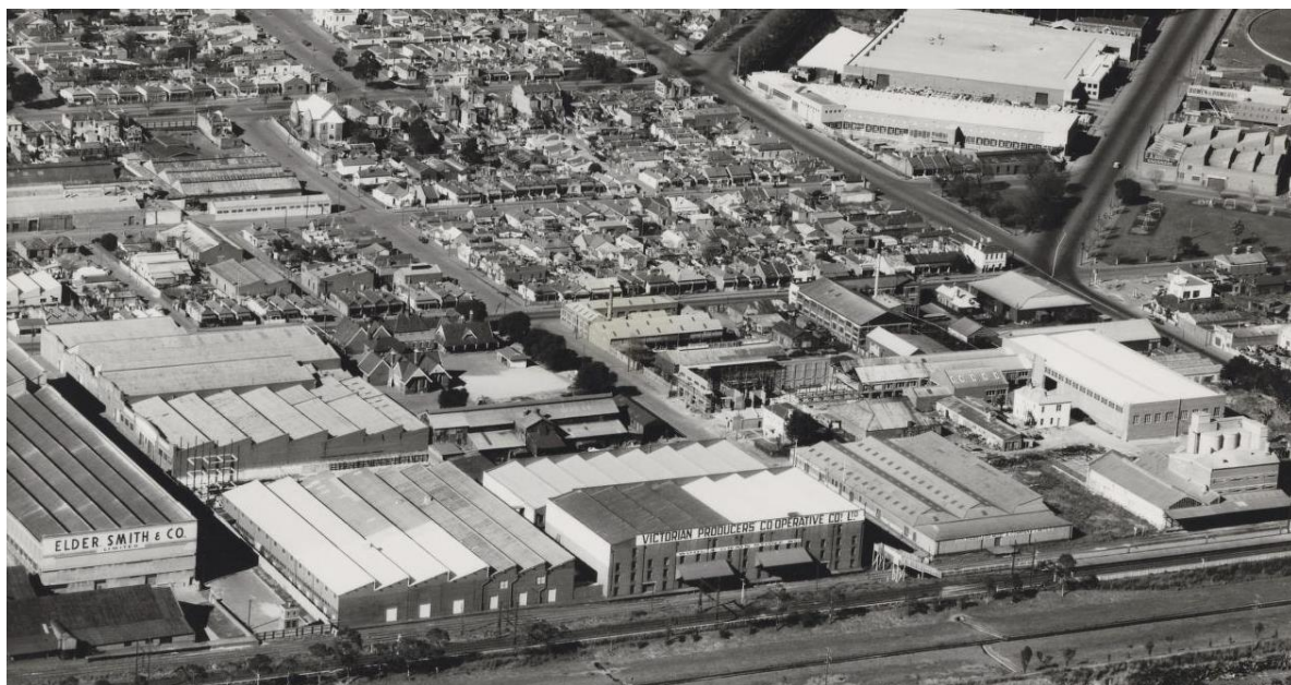
Figure 2.1: Aerial View of North Melbourne – 1950s
