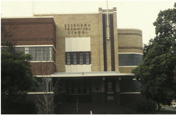
Figure 35: The former Essendon Technical School in Buckley Street, Essendon. Designed by Percy Everett and built in 1938, it is included in the Victorian Heritage Register, H1295 ( http://www.onmydoorstep.com.au/heritage-listing/4929/former-essendon-technical-school )
