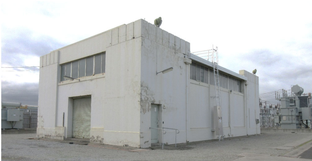
Figure 7: View from southeast on Salmon Street (H Lardner, 09/07/2018)
