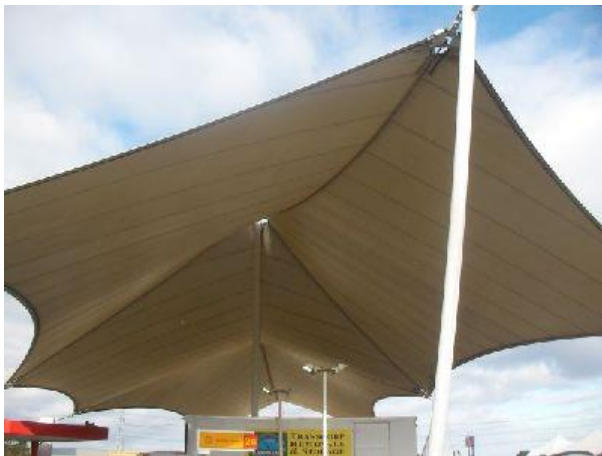
Figure 18: Underside of canopy over the bowzers (Melbourne's Biggest Shade Sail', 1800 Shade U website, https://1800shadeu.com.au/blog/shade-sail-inspector/melbournes-biggest-shade-sail accessed September 2019)
