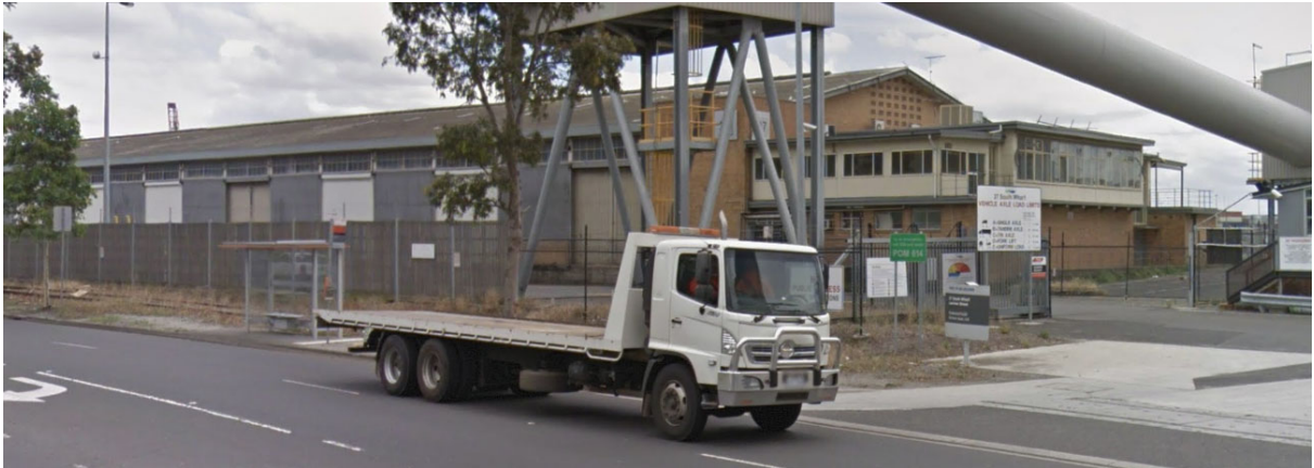
Figure 10: Shed 27, South Wharf at 641-713 Lorimer Street, Port Melbourne (Google imagery December 2017)
