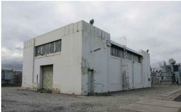
Figure 2: View of the substation from the southwest (H Lardner, 09/07/2018)
