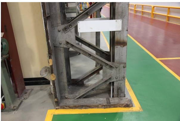
Figure 17: Building 4 column detail (P Mills, 2/5/2018)
