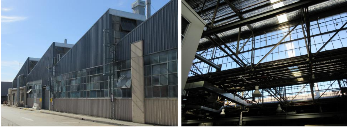
Figures 26 and 27: Plant 3 western side looking towards Bayside Avenue with the medical centre at the far corner, and the interior of Plant 3 illustrating the innovative structural system (HLardner, 18/04/2018)
