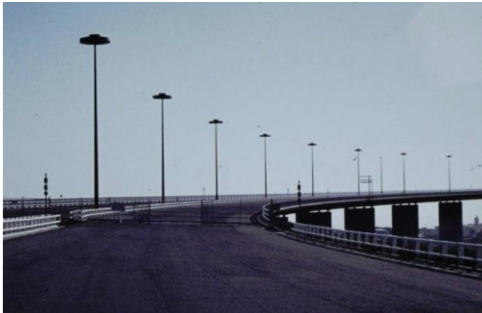
Figure 9: The West Gate Bridge just prior to opening. Note the low side rails and distinctive mushroom-shaped lighting on tall, central stanchions ( https://www.reddit.com/r/melbourne/comments/54dylg/westgate_bridge_pic_during_construction/ )
