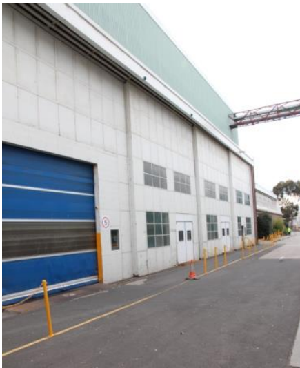
Figure 19: Building 1 hangar doors at eastern corner (PMills, 2/5/2018)
