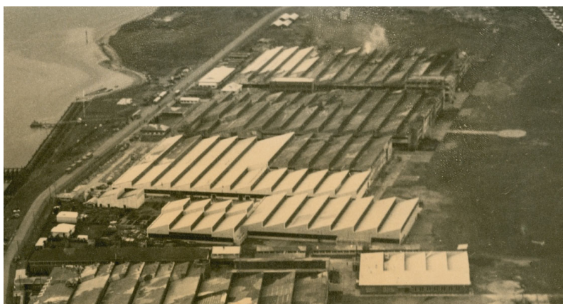
Figure 8: Extract of oblique aerial taken late 1942 or early 1943. No.2 Aircraft Factory has been widened and No.3 Aircraft Factory has been established further to the southwest (Beaufort Division, c1944)
