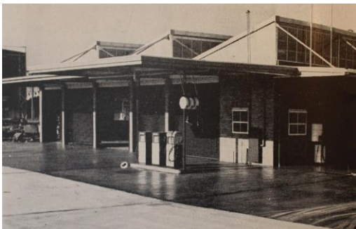
Figure 14: The newly completed garage at the northeast corner of the site, 1961 (Kraftsman, December-January 1960-61)
