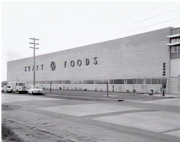
Figure 12: The west side of the production building with a large expanse of brickwork broken by a continuous strip window, c1957. This was soon to be obscured by the 1961-62 addition of a covered loading area (SLV, Acc. No. a42751)
