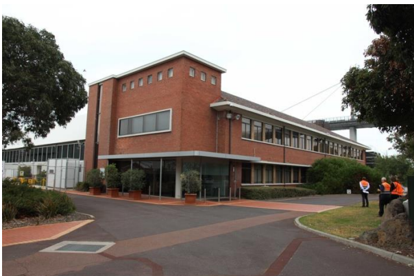
Figure 27: The building 6 frontage (P Mills, 2/5/2018)
