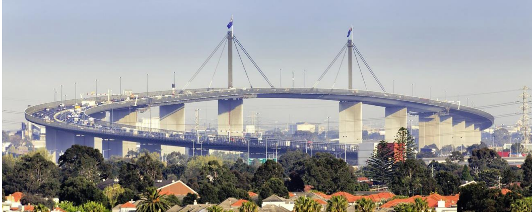
Figure 7: The distinctive curve of the West Gate Bridge and its central pylons with cable stays ( https://www.melbournepoint.com.au/information/west-gate-freeway/ )
