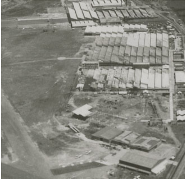
Figure 9: Extract of 1945 oblique aerial showing the new foundry under construction, and the four prefabricated hangars in the foreground. No.3 Aircraft Factory is at top (SLSA PRG 277/143/2)
