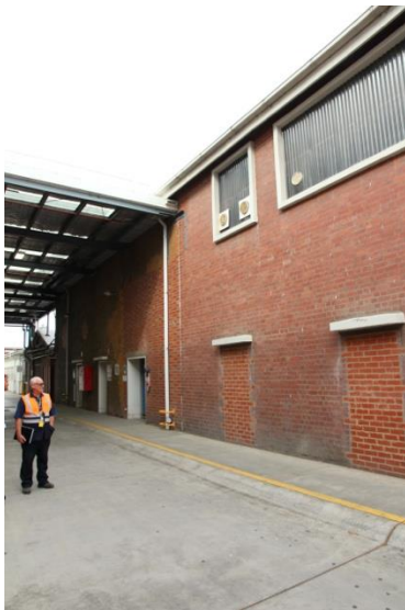
Figure 29: The Building 10 Boiler house from the north (P Mills, 2/5/2018)
