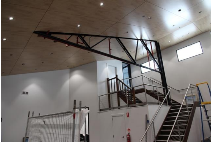
Figure 21: Narrow sawtooth part of Building 1 and stairs to lookout (P Mills, 2/5/2018)
