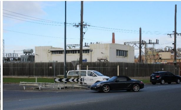
Figure 3: View of the substation from the corner of Salmon and Turner Streets (H Lardner, 09/07/2018)
