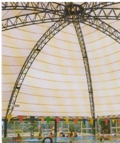
Figure 14: 'Quadome recreational enclosure' at Beaton Park Leisure Centre in Wollongong, 1989 ( W&W , Issue 7 1989, p.3)
