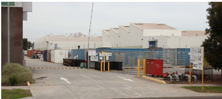
Figure 2: View from Lorimer Street (P Mills, 02/05/2018)
