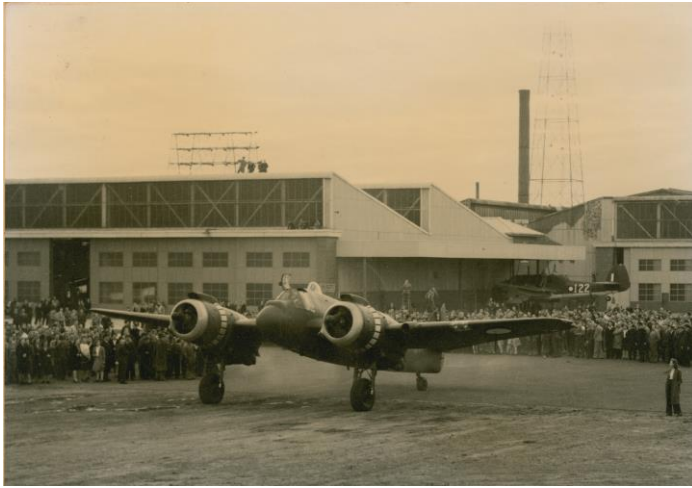
Figure 8: Delivery of the first Beaufighter in mid-1944, showing large double-sawtooth hangar, later to be enlarged, and the infill of the early courtyard on the right (Beaufort Division, c1944)
