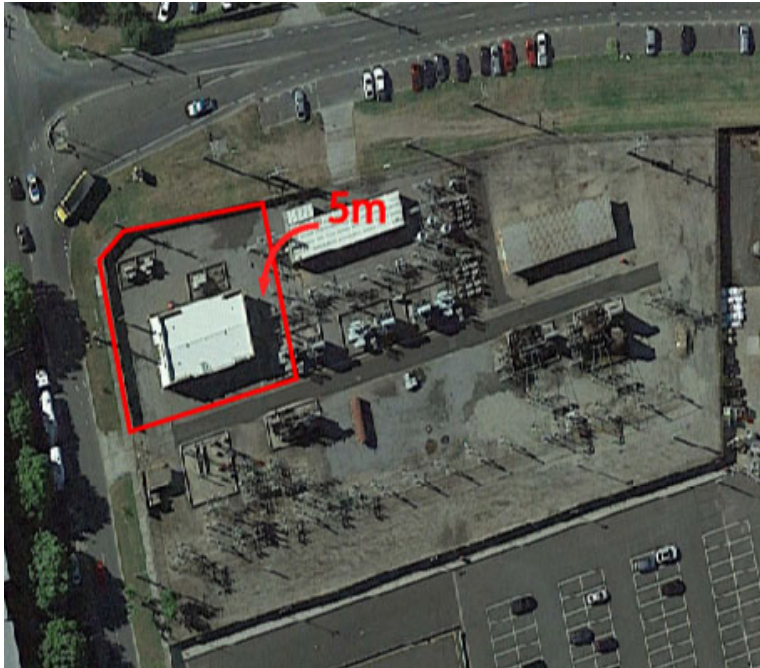
Figure 13: The recommended extent for inclusion in the Heritage Overlay in the Melbourne Planning Scheme.
