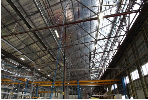
Figure 18: Building 4 interior (P Mills, 2/5/2018)
