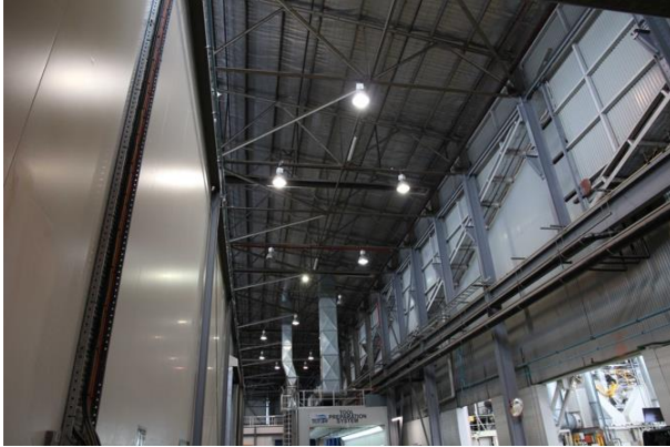
Figure 24: Building 2 interior (P Mills, 2/5/2018)
