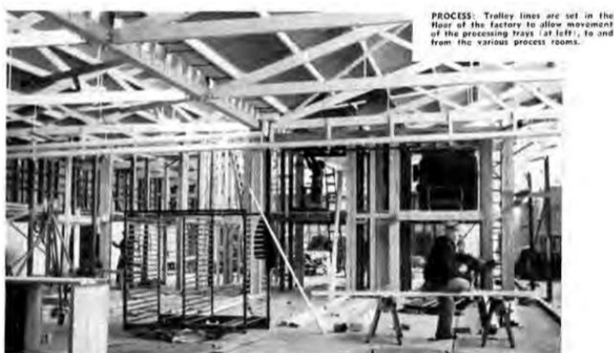
Figure 4: The Fishermans Bend dehydration factory interior under construction in 1943 (Allied Works Council, 1943, p.74).
