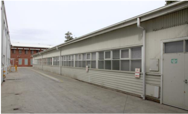
Figure 30: Building 12 as viewed from Avro Lincoln Road (P Mills, 2/5/2018)
