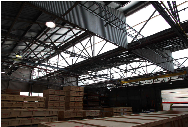
Figure 14: Former No.3 Aircraft Factory interior at the southeast end (P Mills, 2/5/2018)
