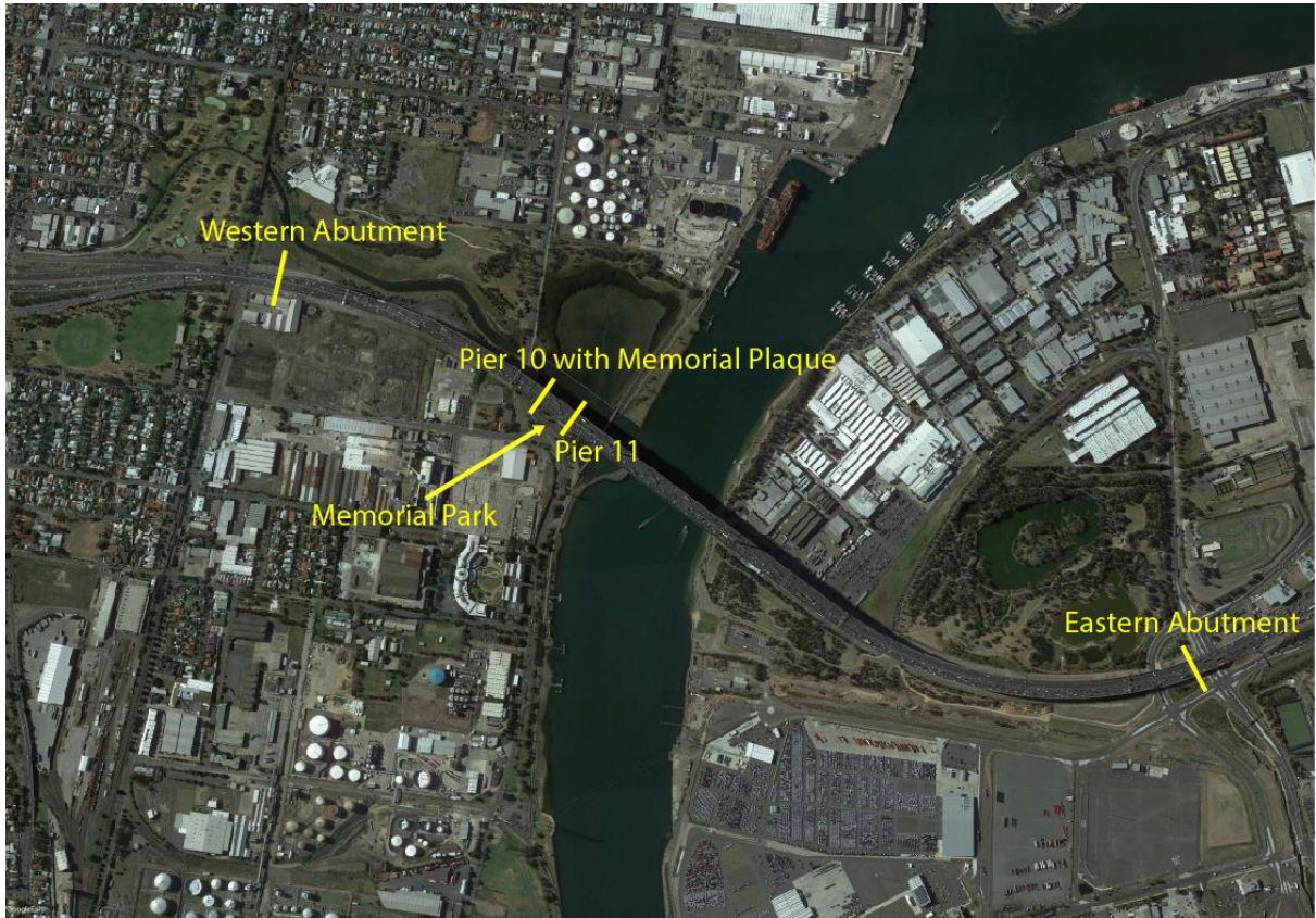
Figure 14: The extent recommended for nomination to the Victorian Heritage Register is the West Gate Bridge between the eastern and western abutments, the Memorial Plaque, and the West Gate Memorial Park
