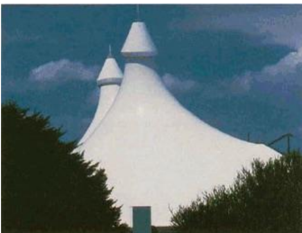
Figure 24: The Keysborough Golf Club driving range roofs shortly after completion ( W&W , 1990 No.8)
