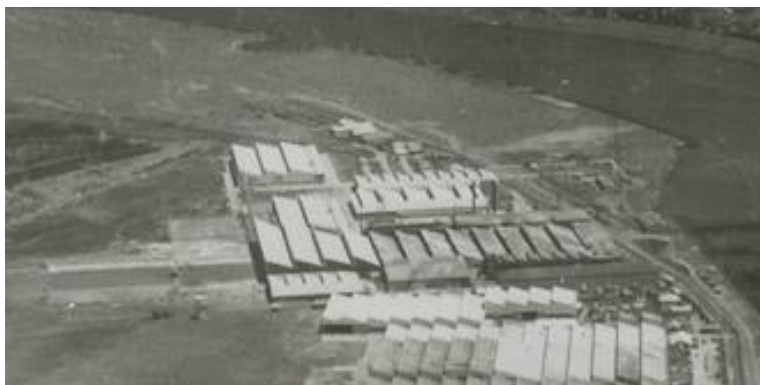
Figure 12: Extract of 1945 oblique aerial showing the second stage of the big hangar (Building 4), joining it with the older main assembly area (parts Buildings 1 and 4) (SLSA PRG, 277/143/2)
