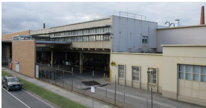
Figure 2: View from Salmon Street (H Lardner, 10/07/2018)
