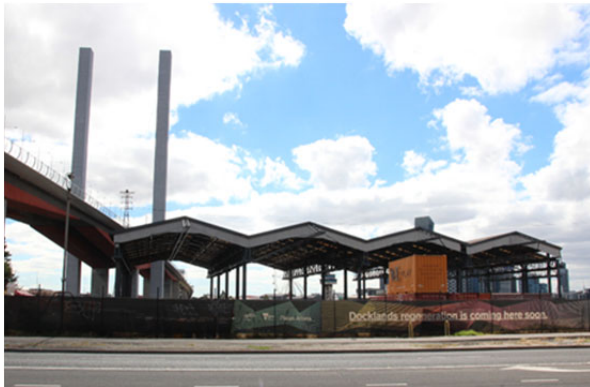
Figure 2: View from Lorimer Street of the 4.5 bays that remain (P Mills, 03/04/2018)
