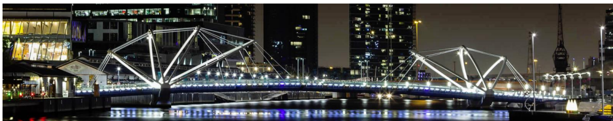
Figure 13: The Seafarers footbridge (2009) is a cable-stayed form like the West Gate Bridge on a much smaller scale ( http://www.fitzgeraldconstructions.com.au/projects/bridge-construction/seafarers-bridge )
