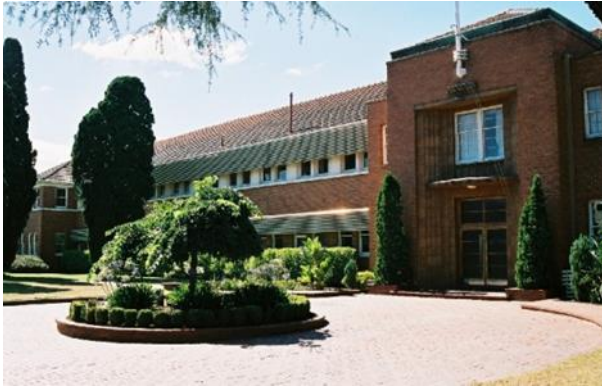
Figure 37: DSTO Administration Building (HLCD, 2004)
