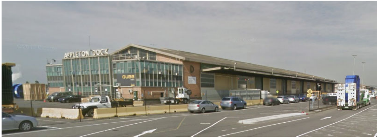
Figure 9: Appleton Dock on Appleton Dock Road, West Melbourne (Google imagery, March 2013)
