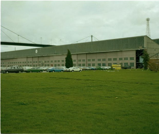
Figure 15: The 600ft (183m) main hangar frontage to the former airfield, GAF / Boeing Buildings 1 and 4, c1978. By this stage part of the former airfield had become a carpark (NAA B6295 6473D0)
