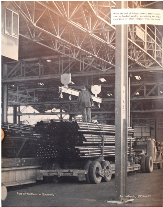
Figure 5: Loading a truck on the south side of the shed, 1958 ( PMQ , January to March 1959, p.14)
