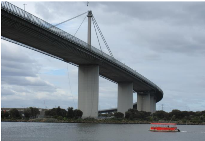
Figure 10: The West Gate Bridge in 2018 after works to strengthen the outer edge for an additional traffic lane and taller safety barriers. (HLardner, 09/07/2018)
