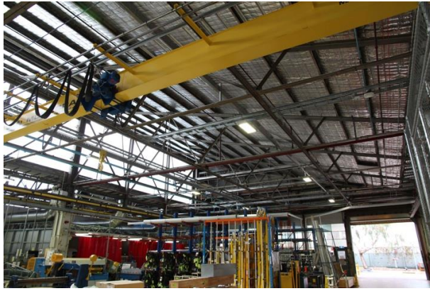
Figure 28: The saw tooth interior of Building 6 (P Mills, 2/5/2018)
