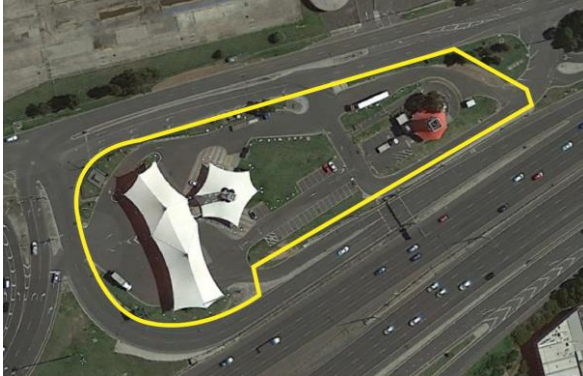
Figure 1: West Gate Service Station North
