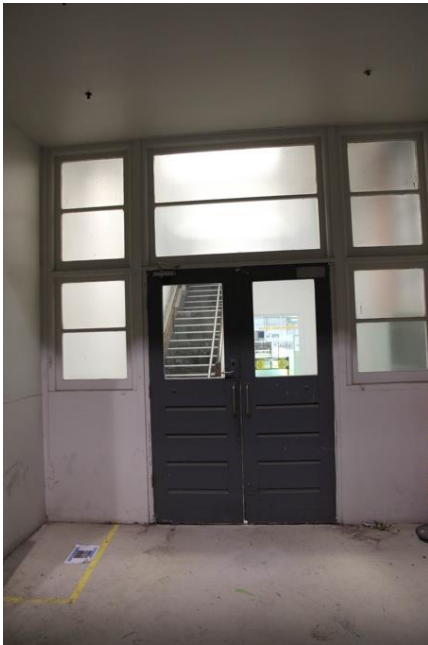
Figure 22: Narrow sawtooth building part of Building 1, and former entry door now in Building 73 (P Mills, 2/5/2018)
