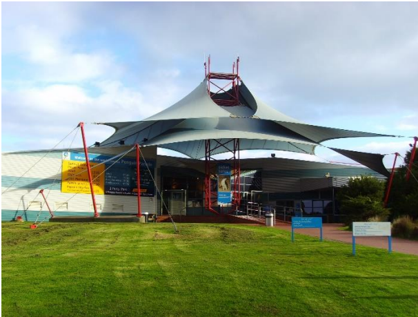
Figure 23: Membrane structure at Penguin Parade Phillip Island (demolished in late 2019) (Gambitek photo, 2006, 'Phillip Island Penguin Parade exterior', Wikimedia Commons website, https://commons.wikimedia.org/wiki/File:Phillip_Island_Penguin_Parade_exterior.jpg accessed September 2019)
