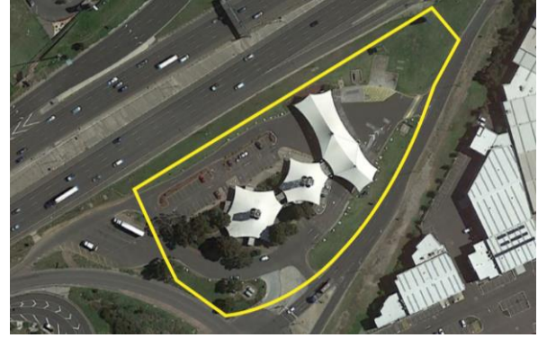
Figure 2: West Gate Service Station South
