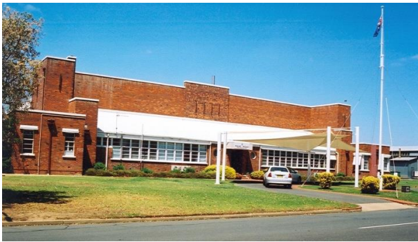
Figure 33: Building 88 Hangar, Wagga Wagga RAAF Base. Built in c1937 by the Commonwealth Department of Works (HLCD, 2003)
