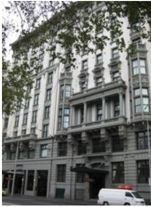
Figure 6. Australian Traveller's Association (now Rendezvous Hotel) constructed 1912.
