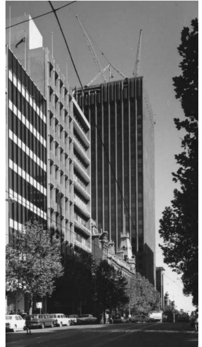
Figure 1 - AMP Tower under construction in 1969
