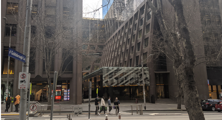
Glass canopy - plaza access from Bourke Street
