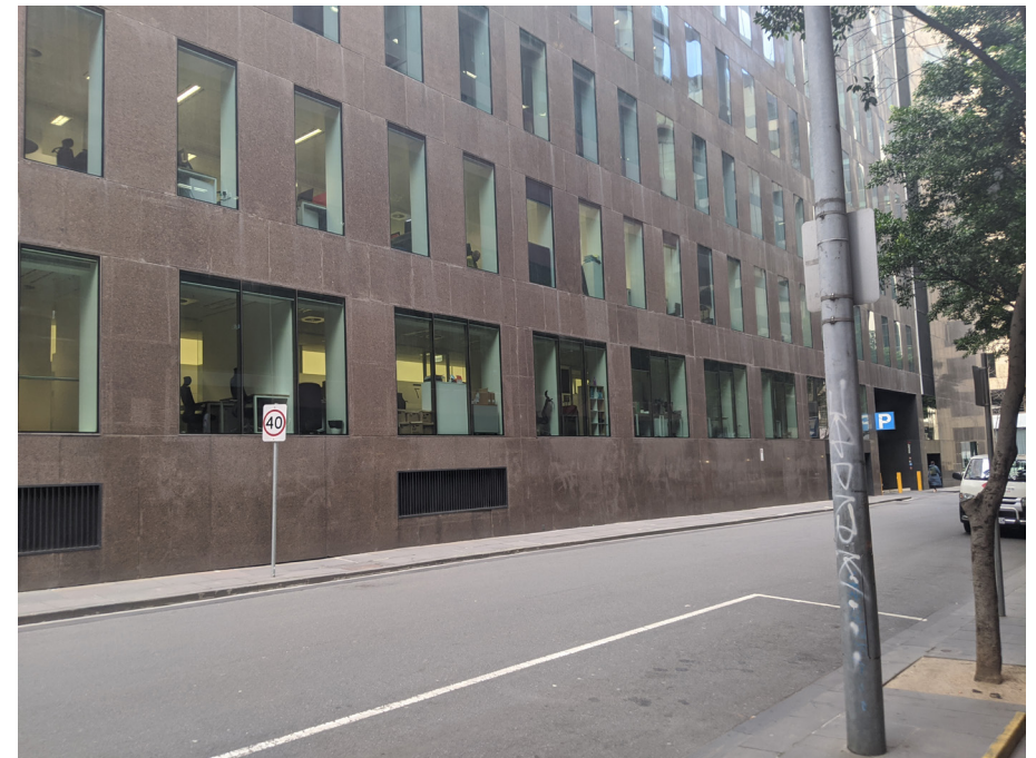
Figure 13 - St James Building frontage to Church Street
