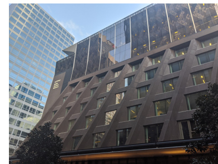
B & H - Additional levels on St James Building
