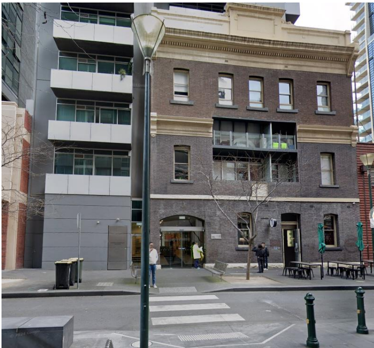
Figure 11 25-29 Wills Street, Melbourne (Source: Google Maps accessed 4/6/25)
