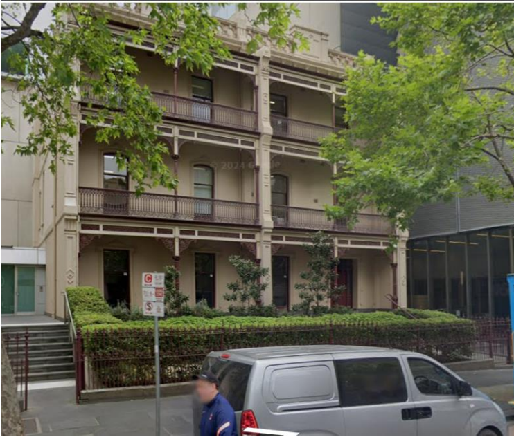
Figure 9 Streetview image of 472-474 Lonsdale Street, Melbourne (Source: Google Streetview via CoMPASS accessed 2/6/25)
