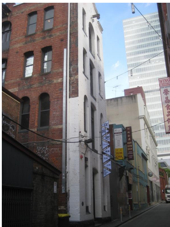
Figure 14 11 Heffernan Lane, Melbourne (Source: CoMPASS, accessed 11/6/25)
