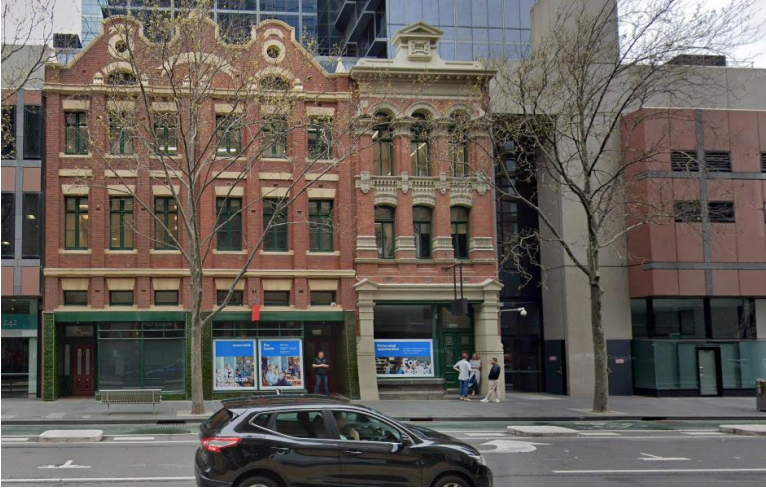
Figure 5 Heritage fabric at 266-272 Exhibition Street, Melbourne (Source: Streetview via CoMPASS accessed 11 June 2025)
